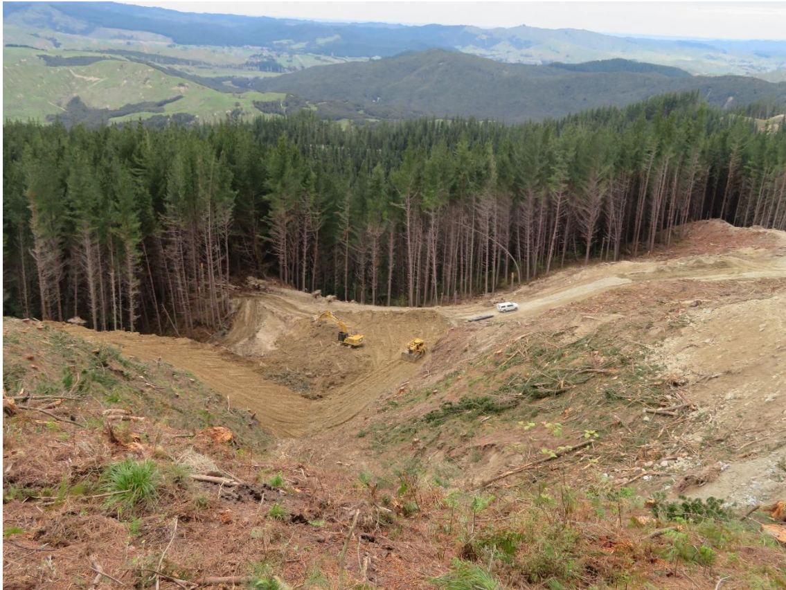
Photo 1: Construction of Zuberi Rod from Landing 909 to temporary landing.
