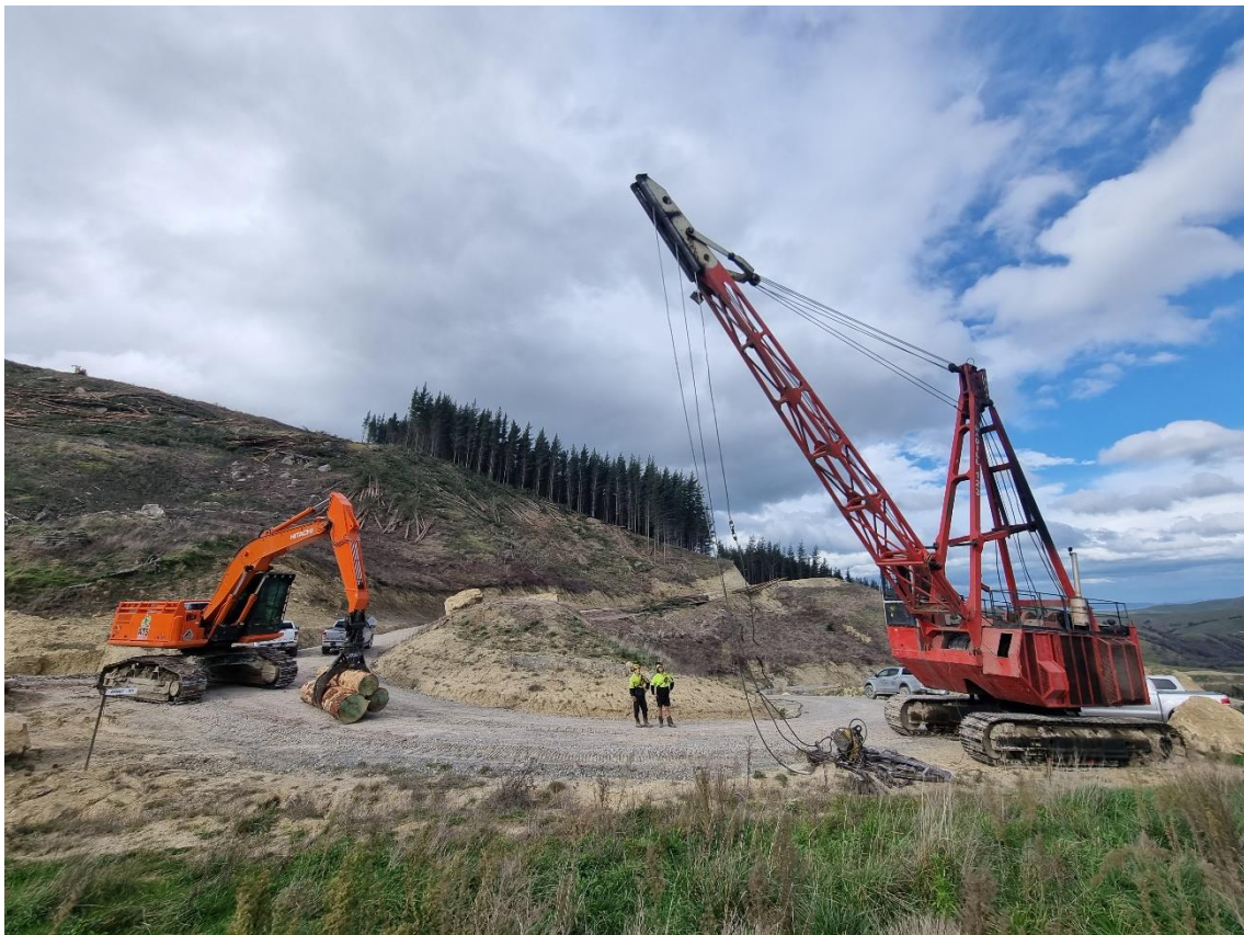
Photo 8: Machine fixed and ready to get back to work.
