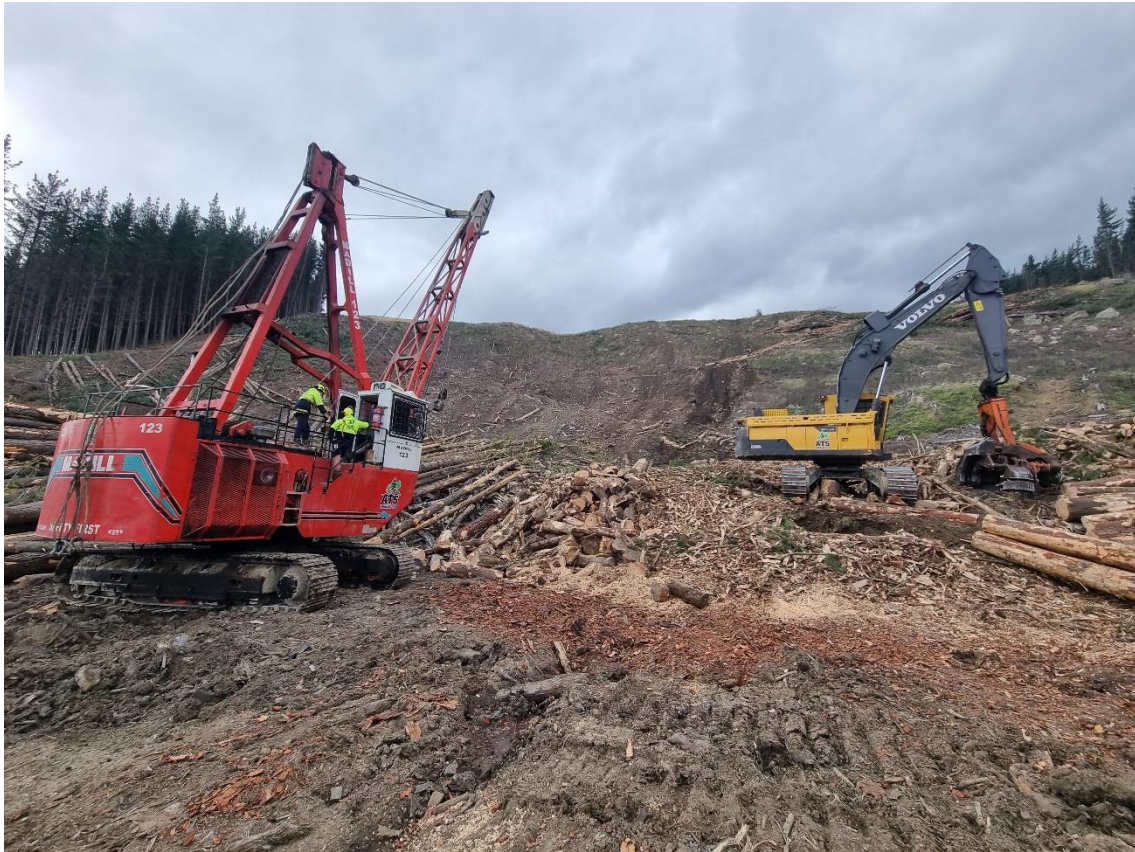
Photo 7: Swing yarder back in place ready to be anchored down.
