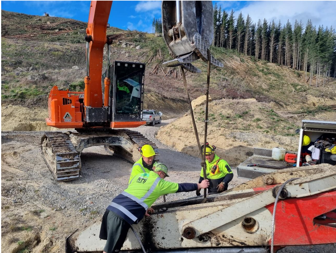
Photo 9: Loader helping to lift a wheel to remove a broken bearing.
