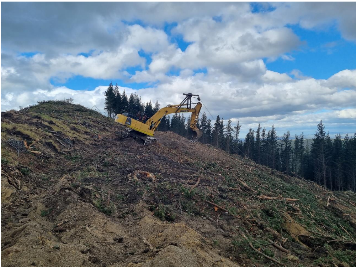
Photo 4: Tail hold machine moving to give best deflection for cables.
