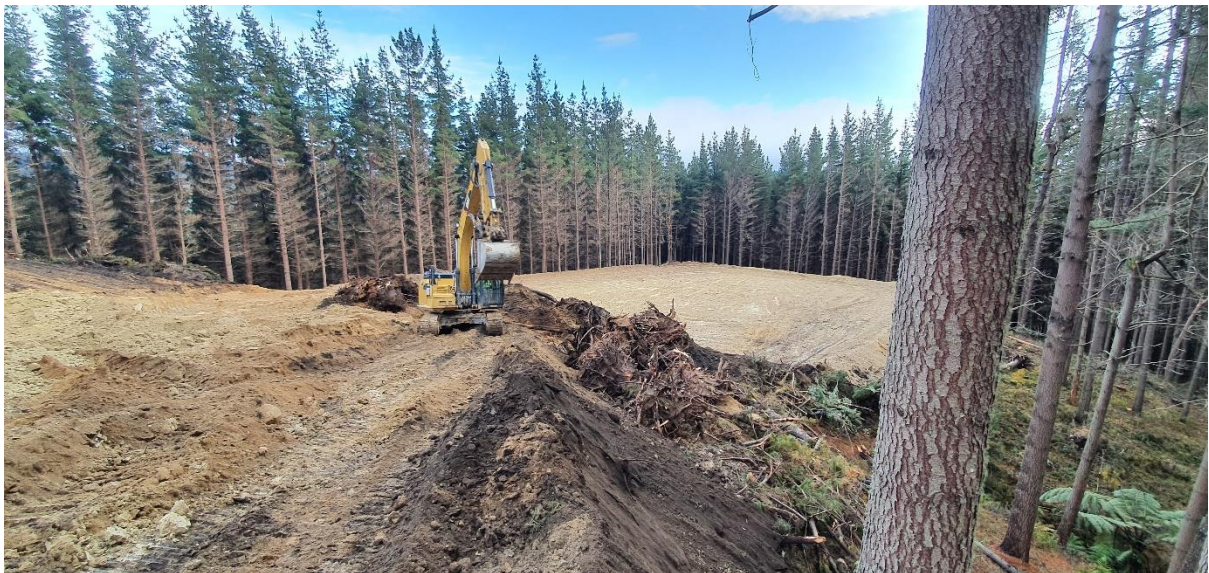
Photo 4: Earthworks on Landing 119.
