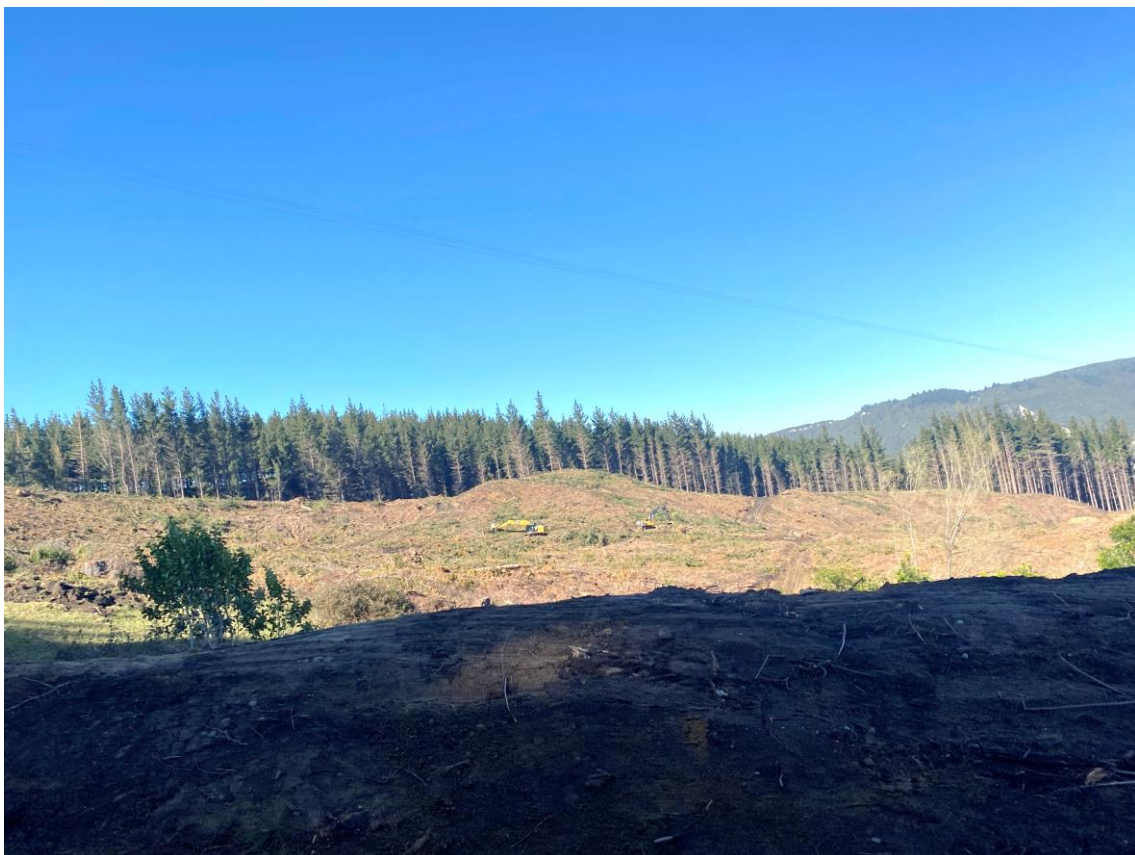
Photo 2: Galbraith Earth Movers rehabbing haul tracks in Setting 4.
