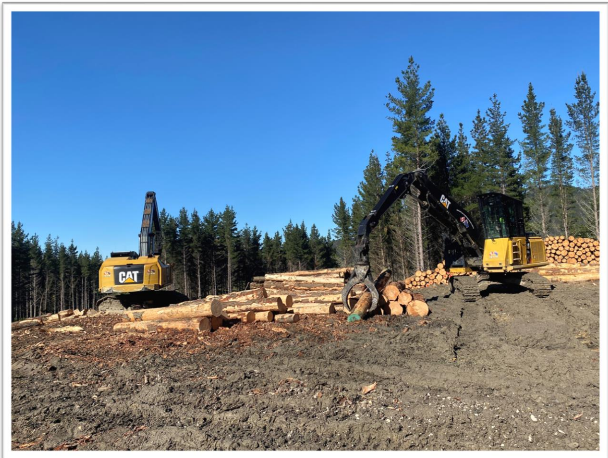
Log 17 processor and log loader working on Landing 11.
