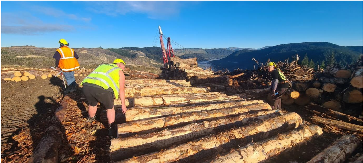
Photo 4: Quality control on Landing 24.
