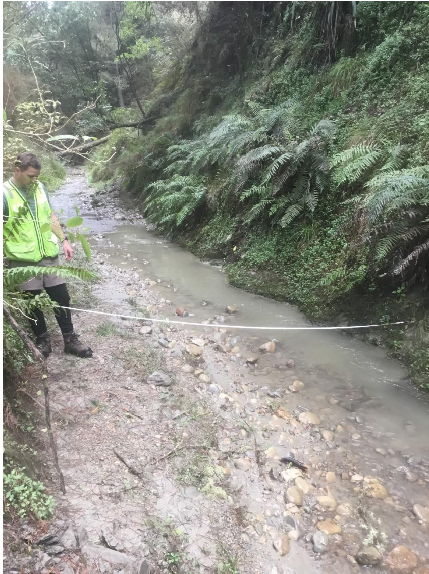
Photo 1: FMNZ measuring stream for river crossing design.
