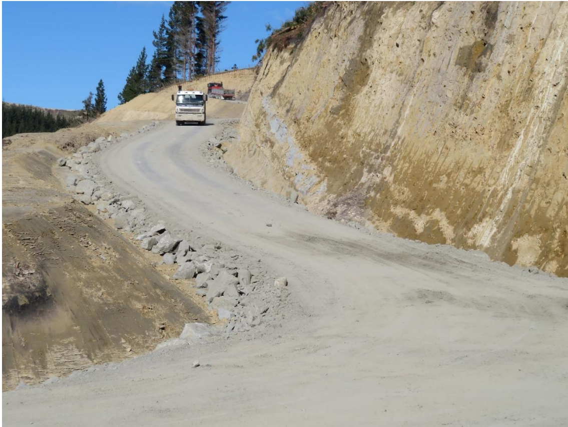
Photo 7: McCoy Road from Landing 101A to 101B.
