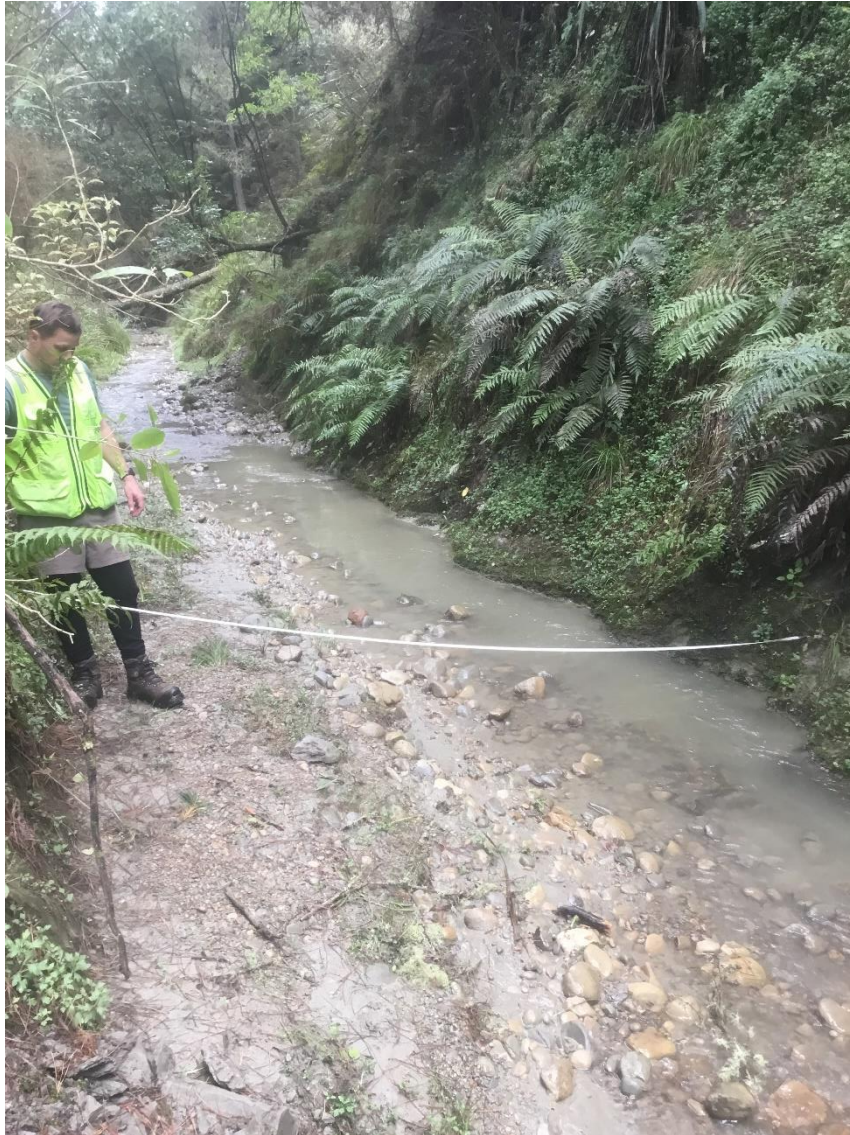
Photo 1: FMNZ measuring stream for river crossing design.
