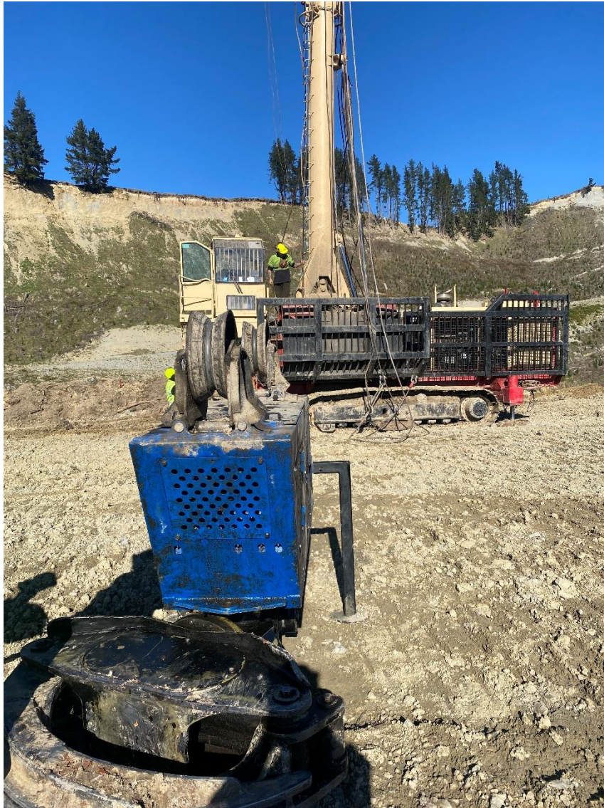
Photo 4: Log 11 hauler being set up on two-stage Pad 18A with grapple carriage in foreground.
