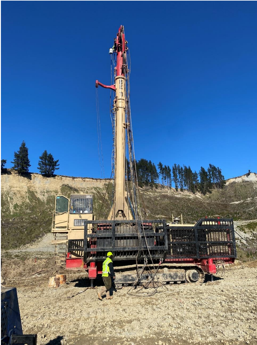
Photo 5: Log 11 hauler being set up on two-stage Pad 18A.
