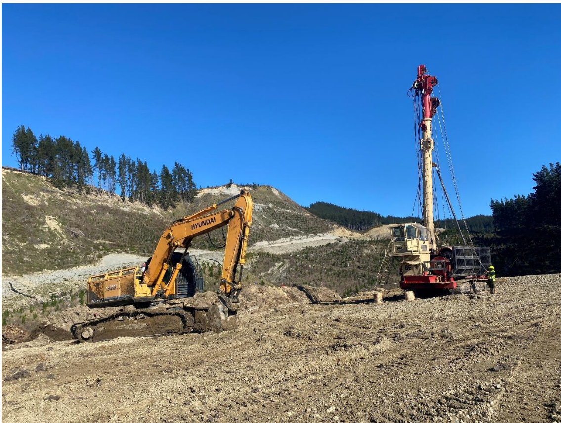
Photo 2: Pole hauler setting up on Landing 18.
