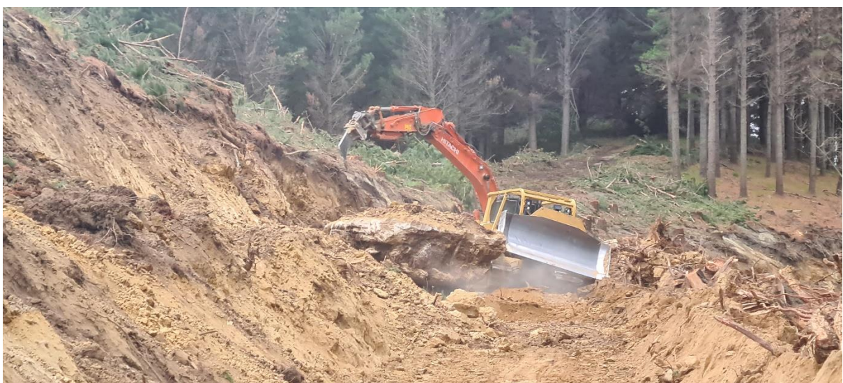
Photo 3: Clearing a large boulder to construct Tutaekuri Road to Landing 29.
