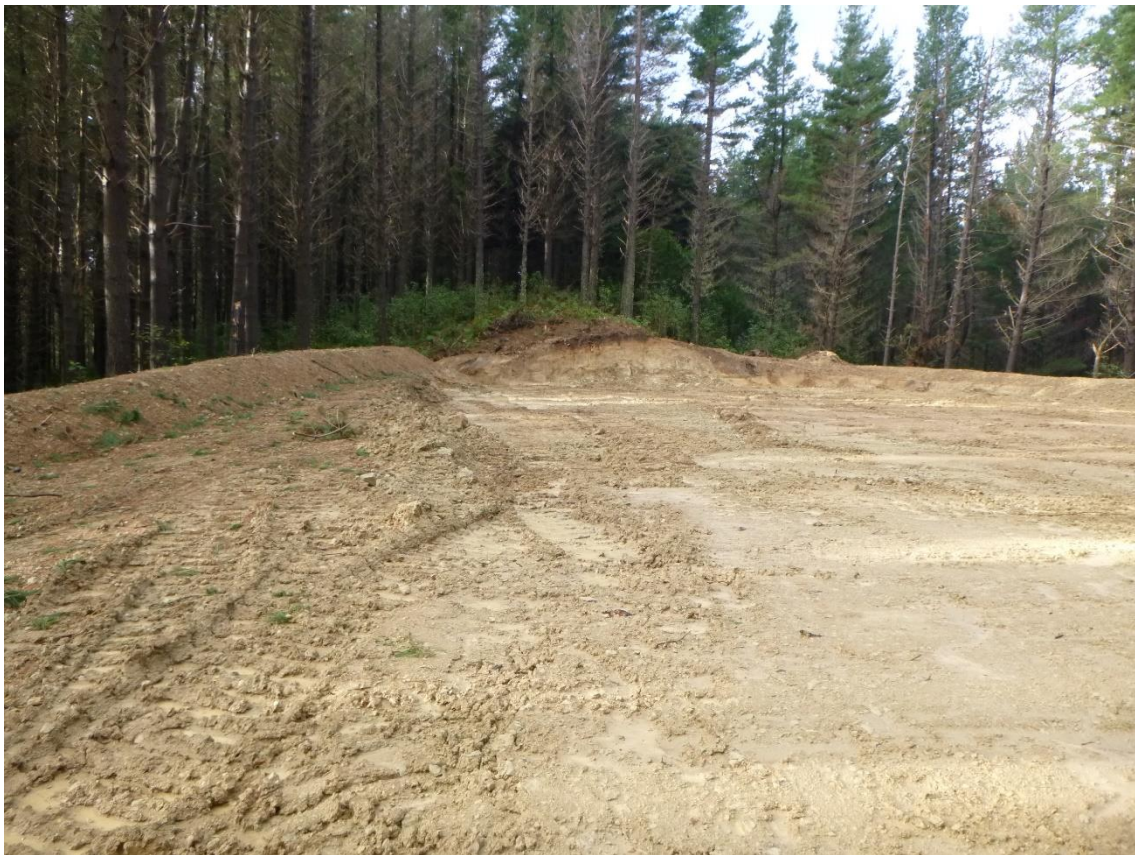
Photo 2: Tahurua Earthmovers – enlarged Pad 16 at the end of Dixon Road.
