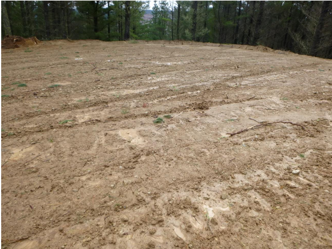
Photo 1: Tahurua Earthmovers – completed formation of Pad 15 at the end of McIntosh Road.
