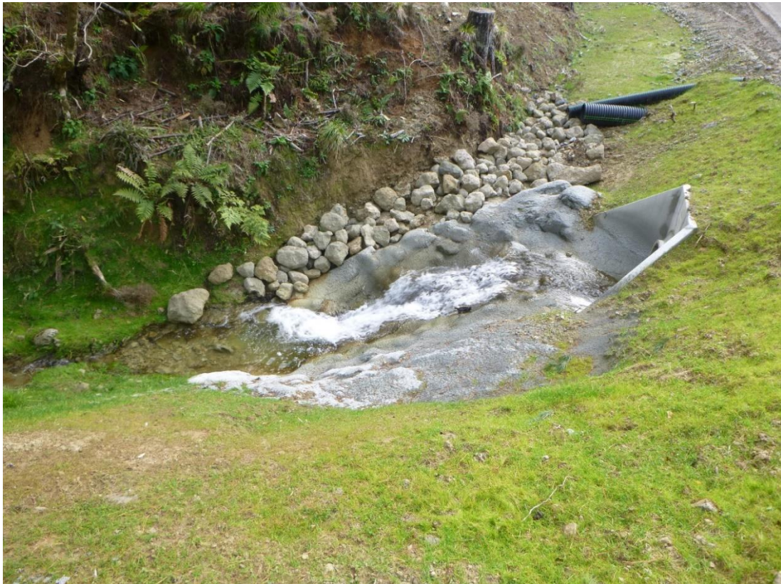
Photo 4: Water exiting Crossing 4 on Rolfe Road with fish passage maintained on the concrete ramp, and strong grass growth following seeding.
