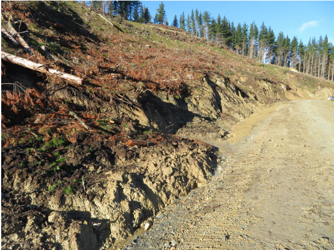
Photos 1 & 2: Batter slump post weather event, Landing 314.
