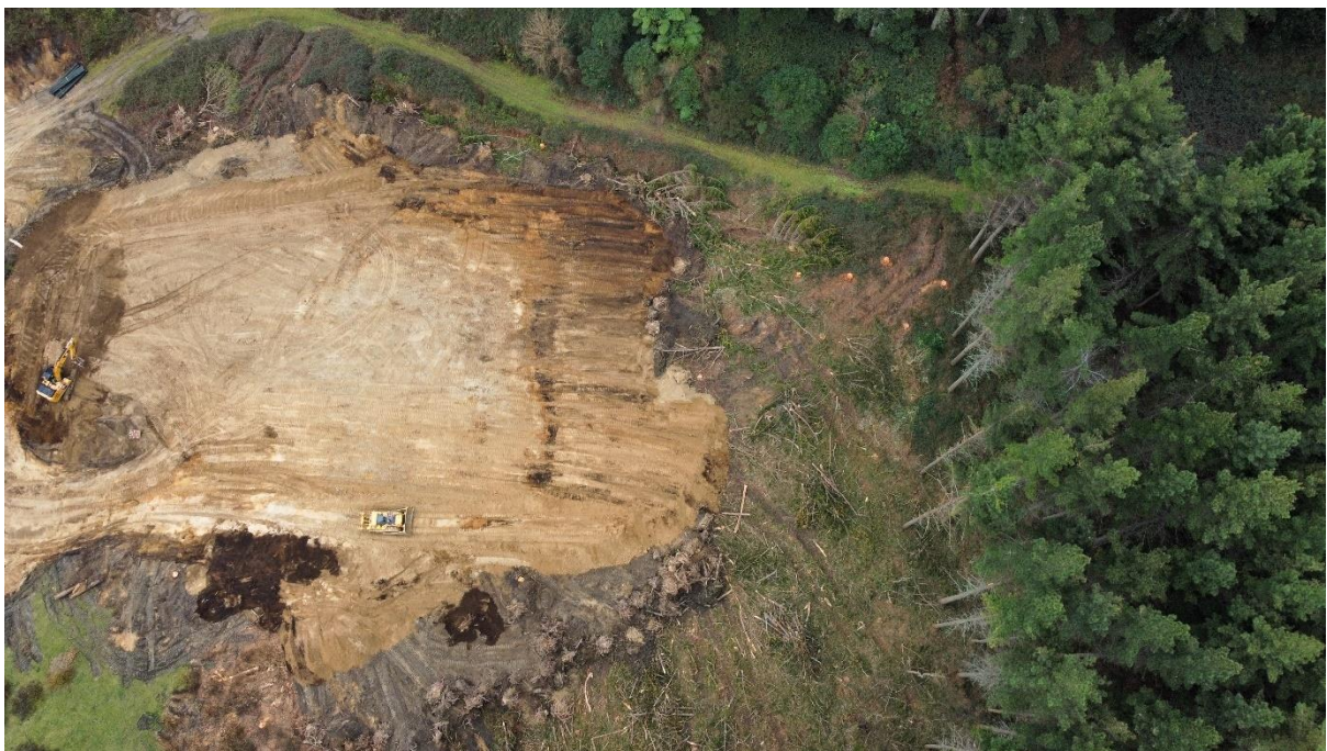
Photo 2: Drone photo showing Galbraith Earth Movers constructing Landing 6.
