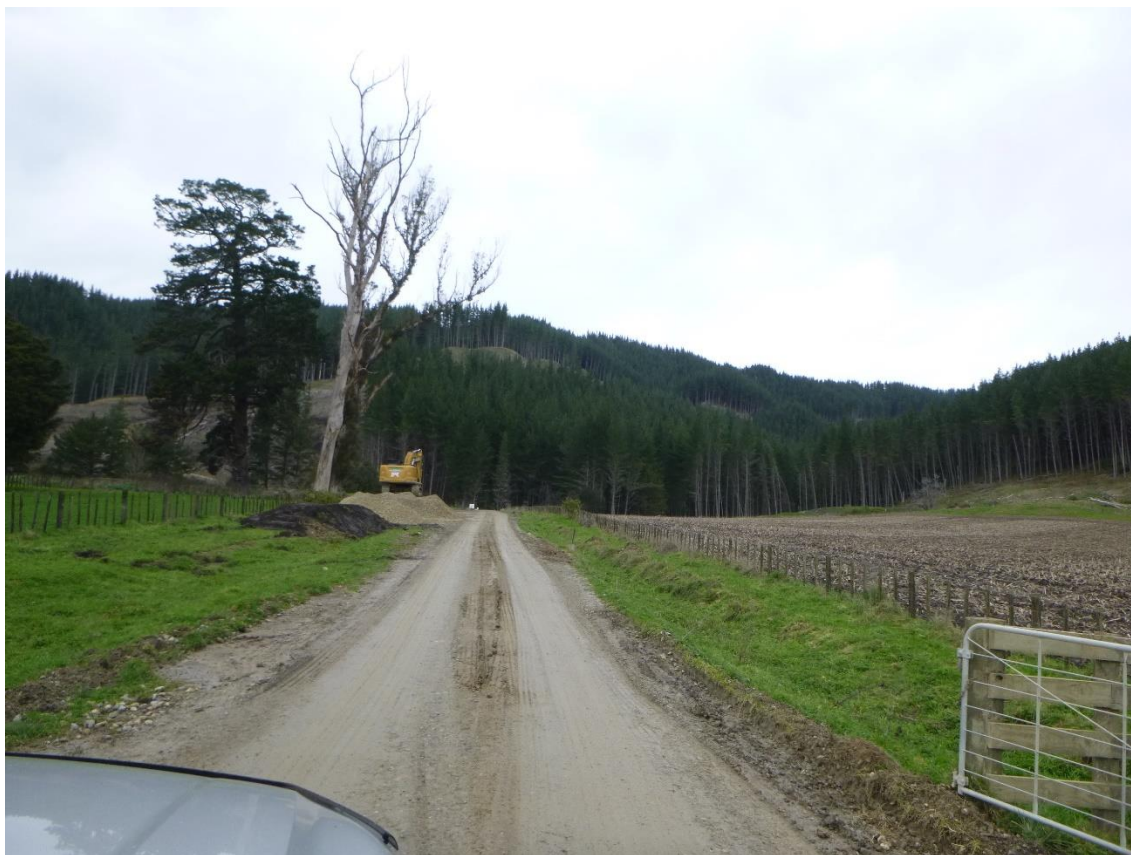
Photo 1: Richmond Road easement, aggregate stockpile for off load when access to the top is difficult in wet weather.
