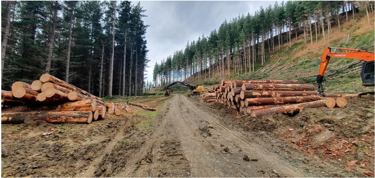
Photo 5: Log 58 daylighting Elliott Road, Landing 103.
