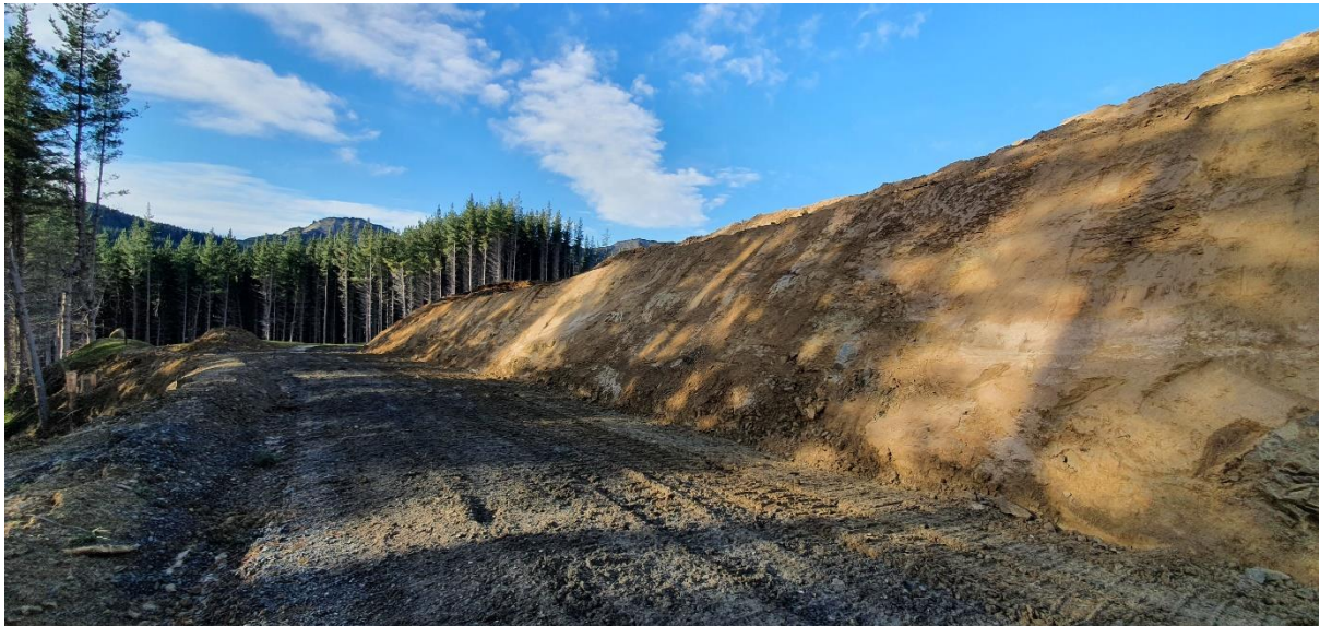
Photo 6: Repairs to Bushmills Road.
