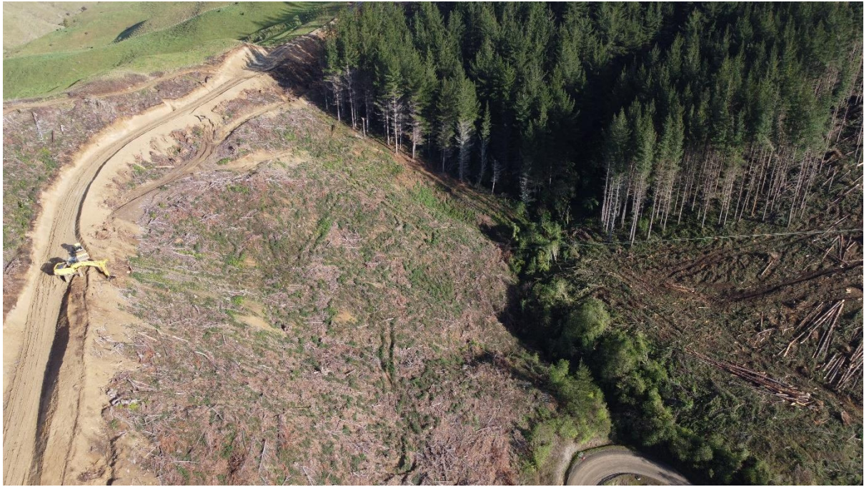
Photo 3: Backline machine on Adams Road supporting the ropes for the harvestline in Setting 132.
