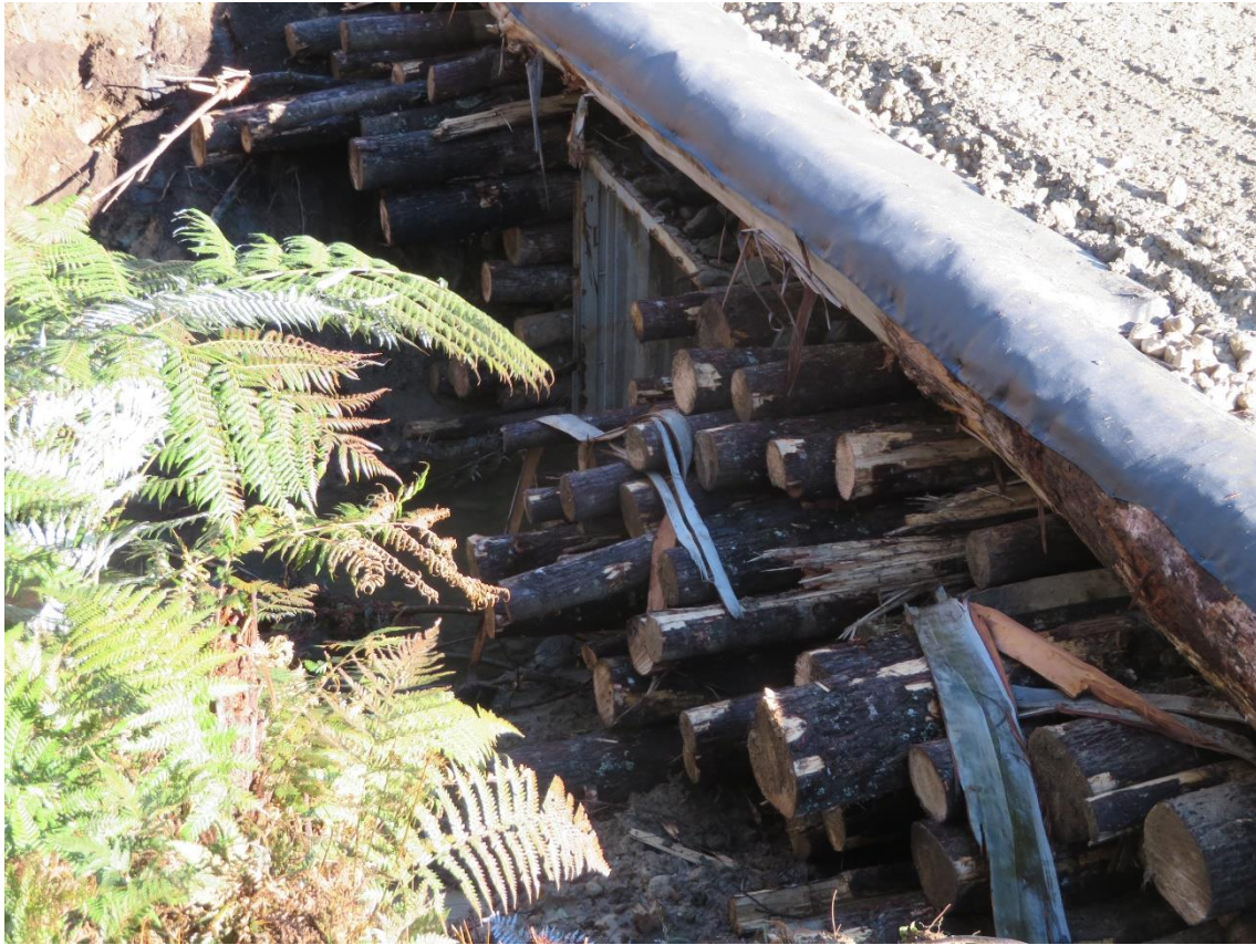
Photo 7: Poplar logs around temporary container crossing.
