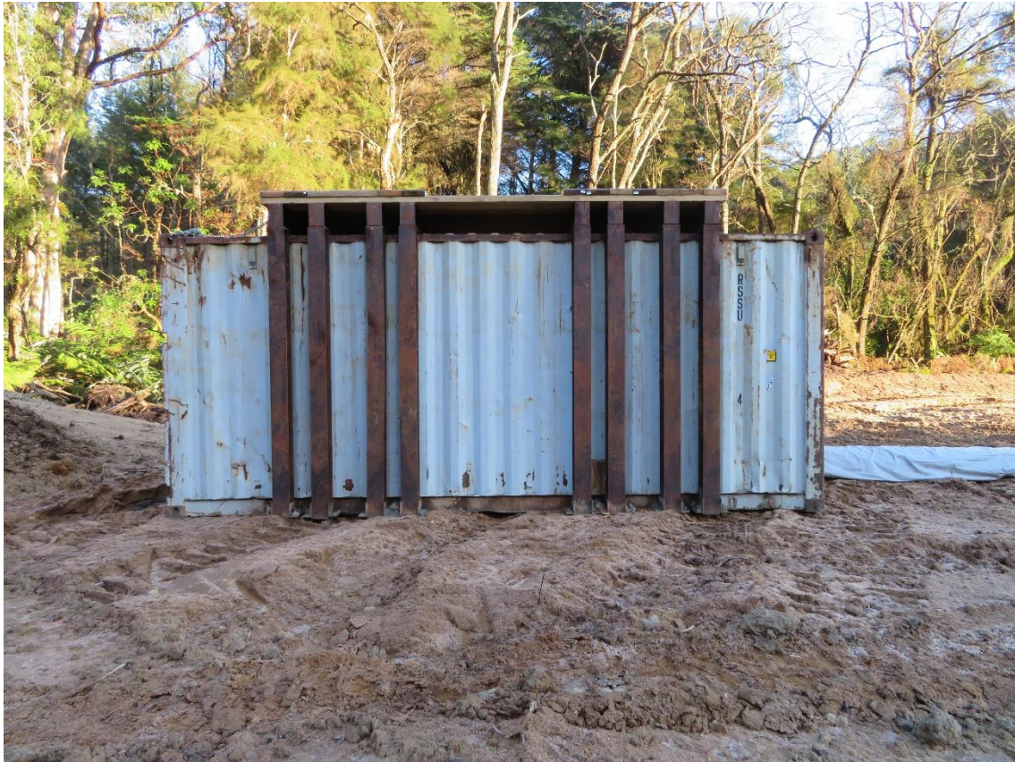
Photo 5: Container for the temporary crossing.
