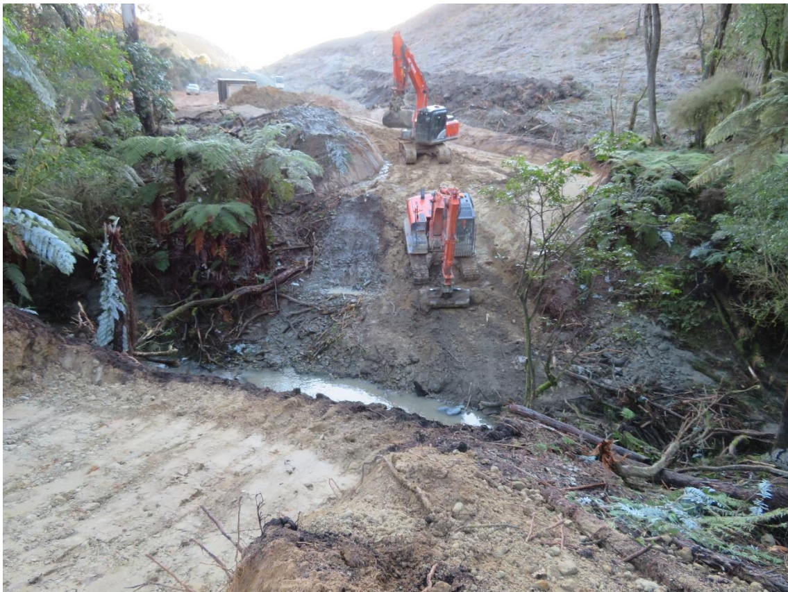
Photo 4: Temporary crossing preparation.
