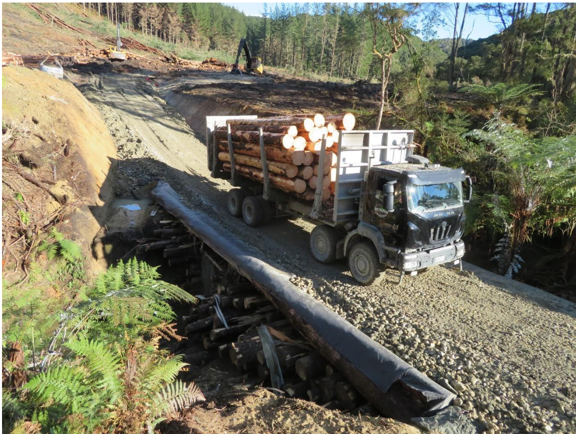
Photo 8: Staging truck going across temporary container crossing.
