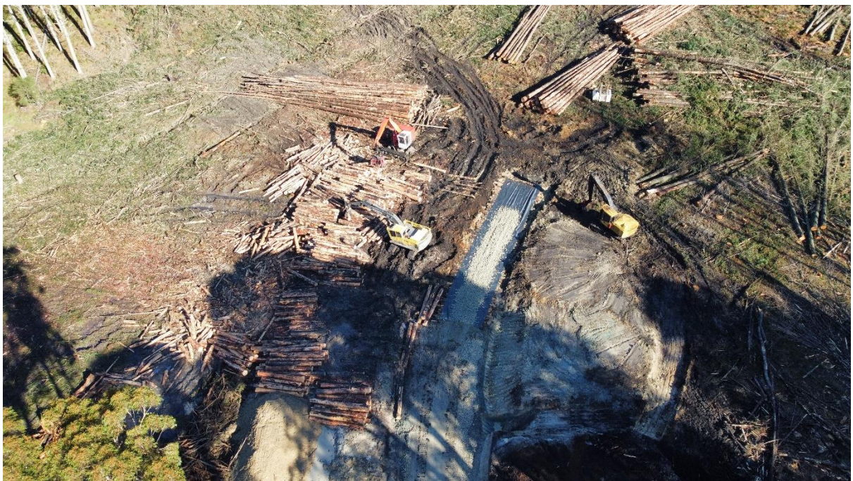
Photo 2: Roadline processing site.
