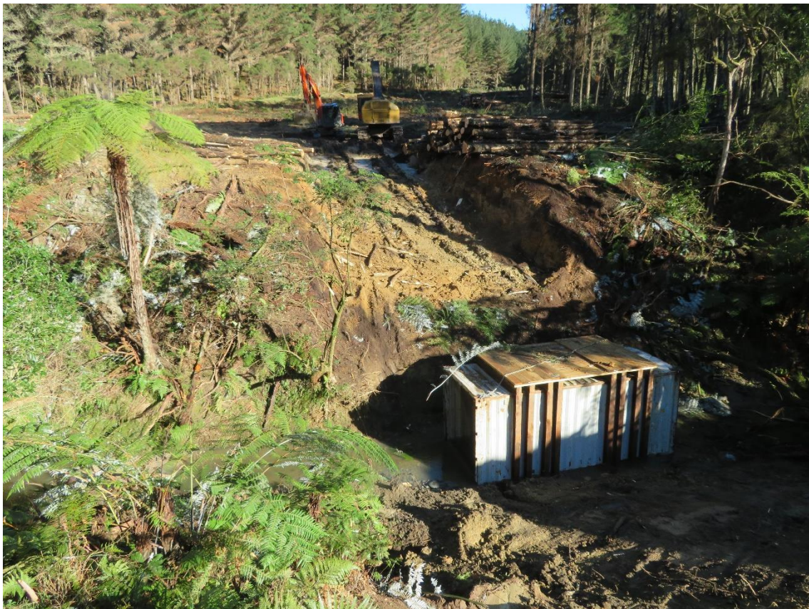
Photo 6: Container in place for the temporary crossing.
