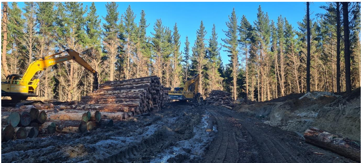
Photo 5: Logs from roadline on Siobhan Road awaiting loadout.
