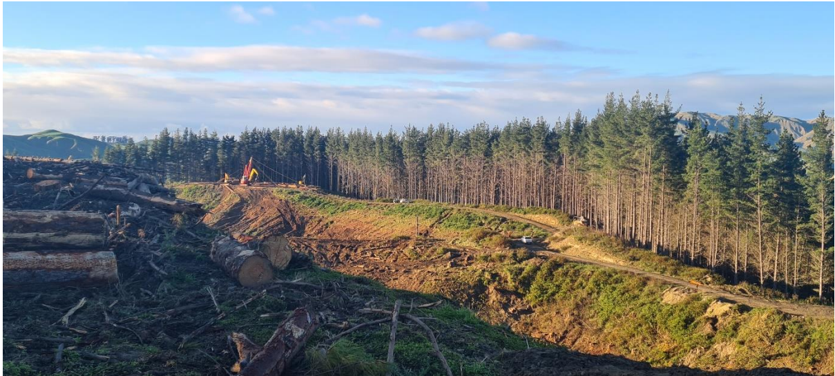
Photo 1: Swing yarder on Landing 19 pulling Settings 17 and 18.
