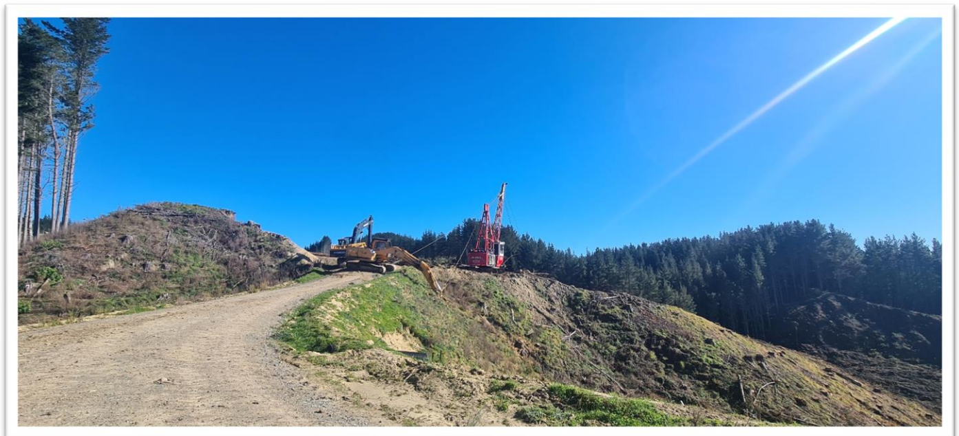
Swing yarder on Court Road pulling Setting 18.
