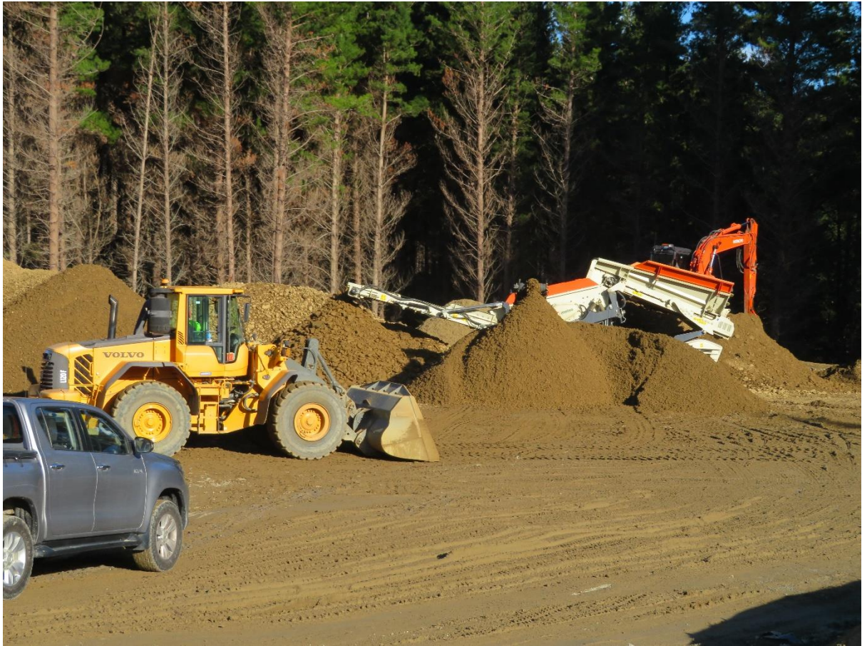
Photo 8: Screening overs from red metal. "Overs" are the larger rocks which are being separated (screened) from the finer rocks.
