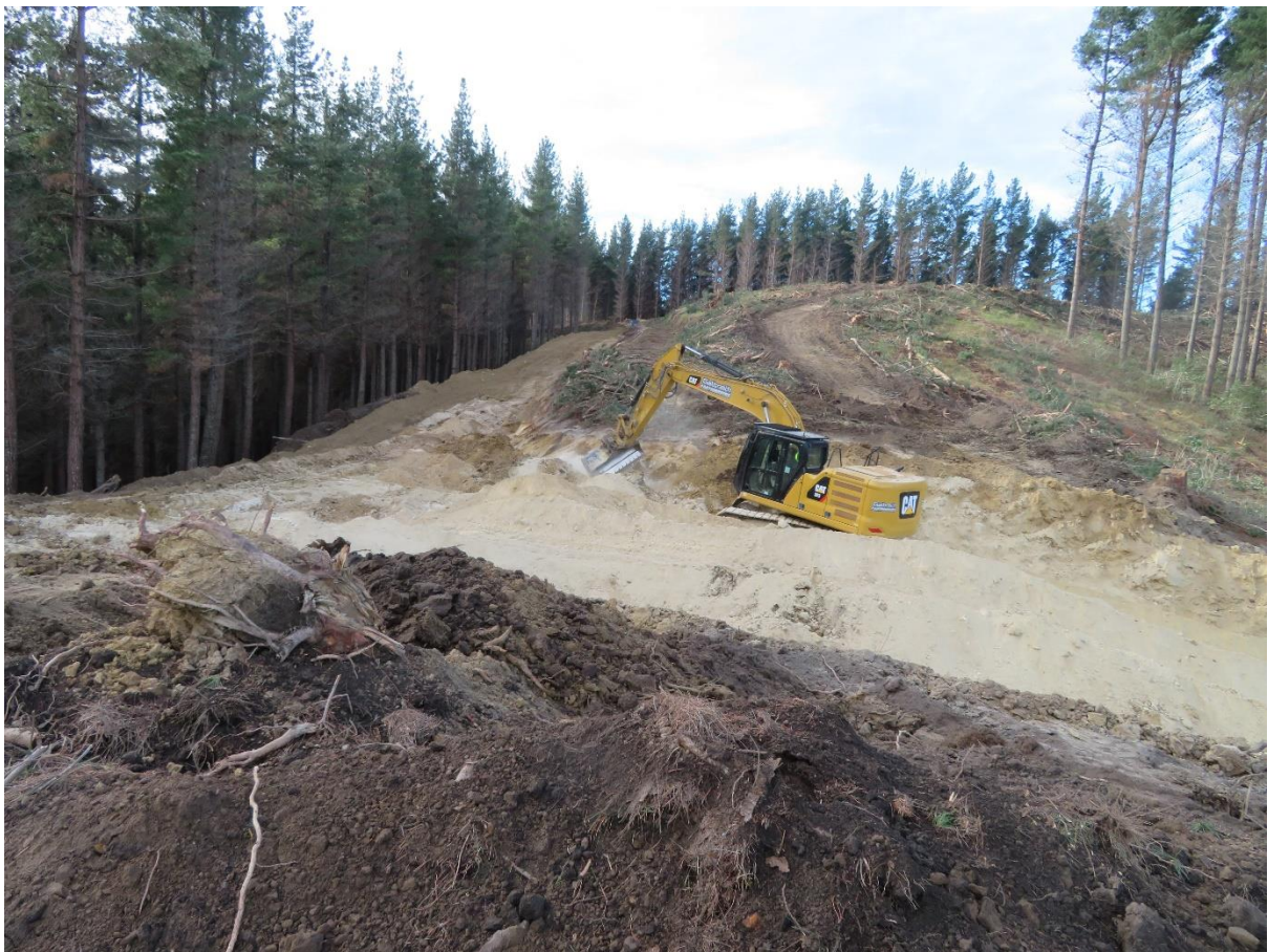
Photo 5: Faulkner Road, construction of Landing 13.
