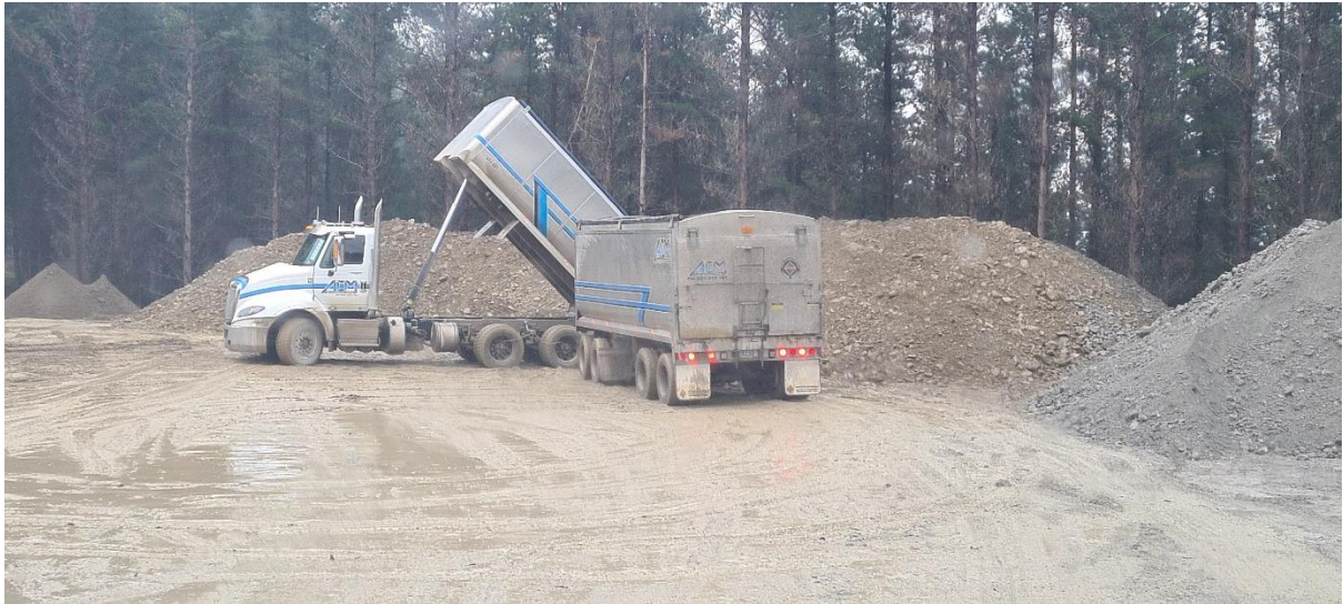
Photo 1: Metal being delivered for Tutaekuri Road.
