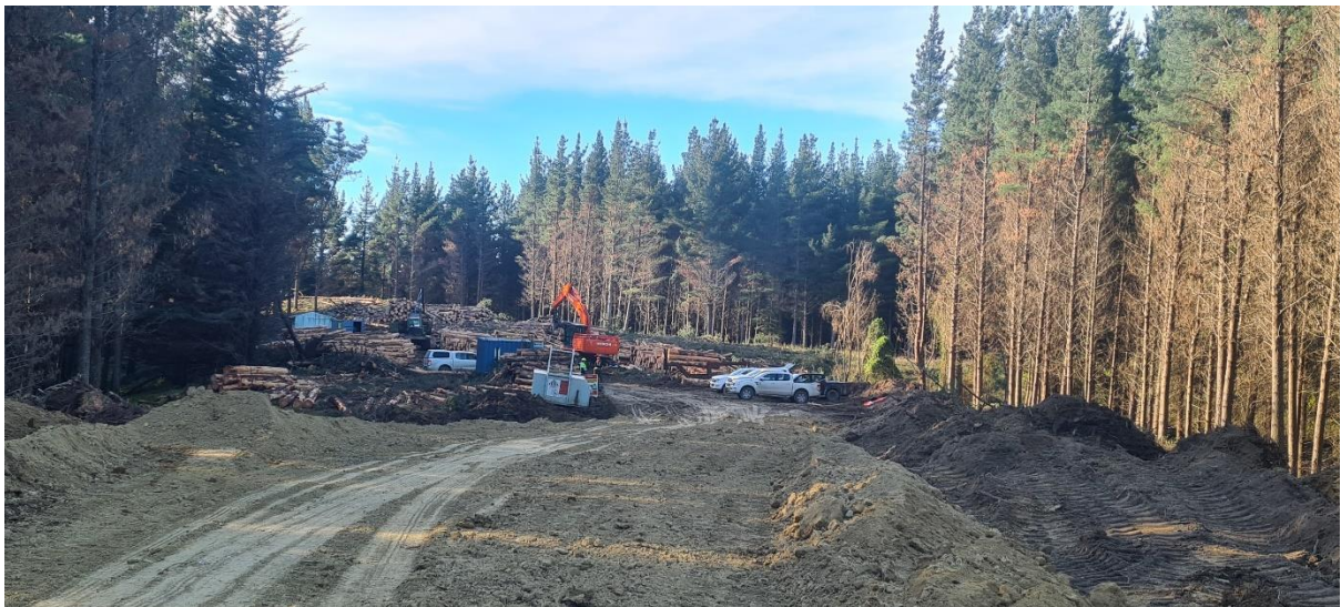
Photo 7: Log 8 on Landing 27, Tutaekuri Rd.
