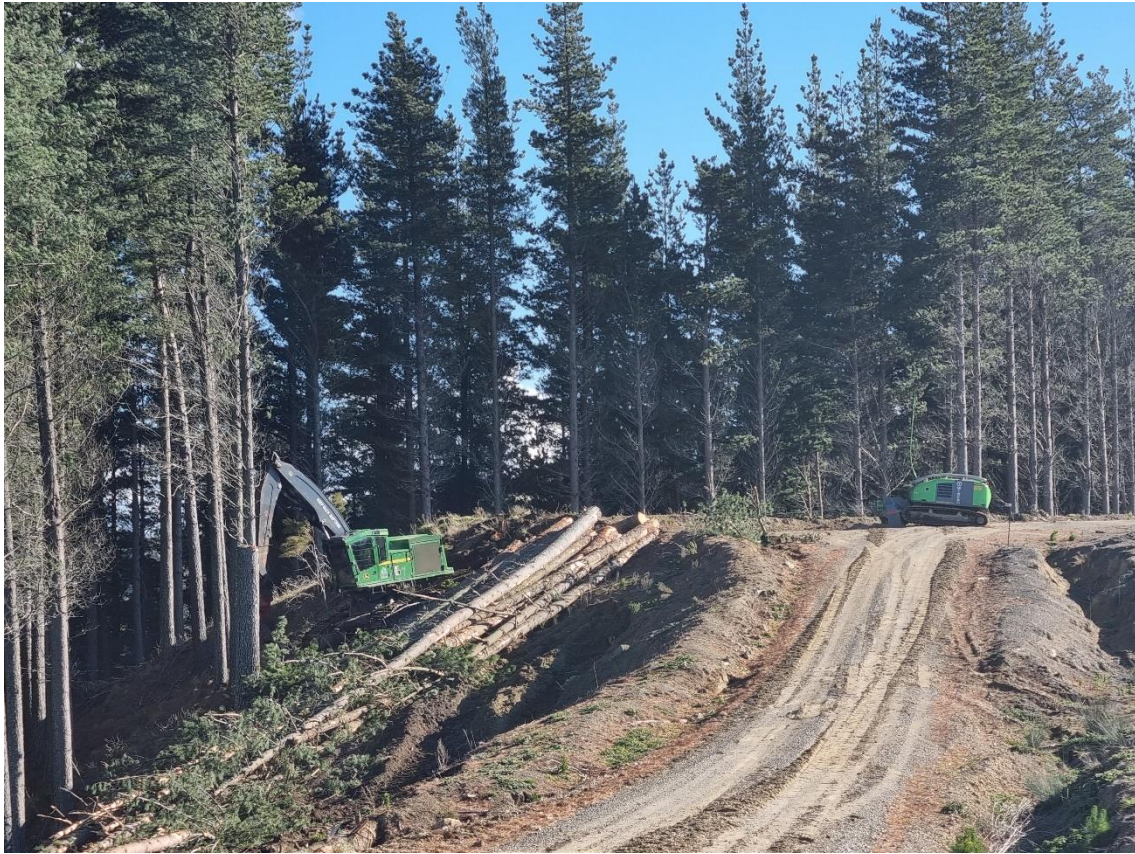
Photo 9: Tethered assisted machine feller going over a steep face.
