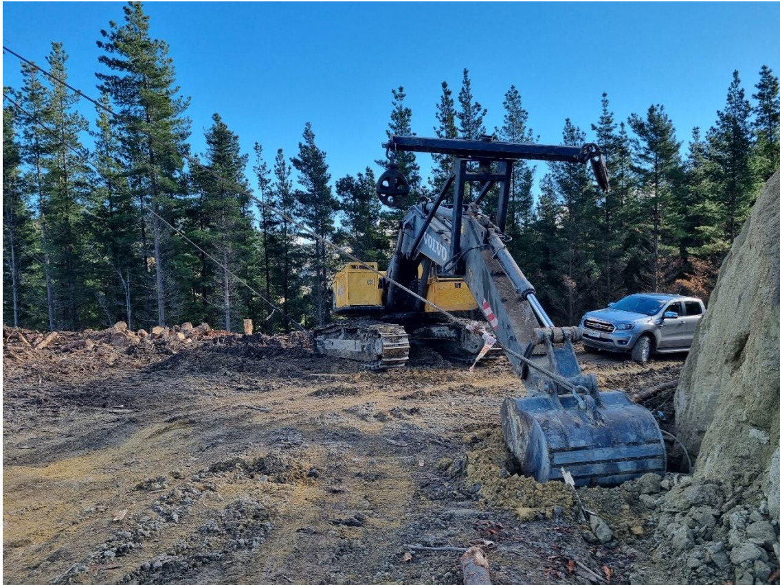
Photo 7: Anchor ropes held down by machine.
