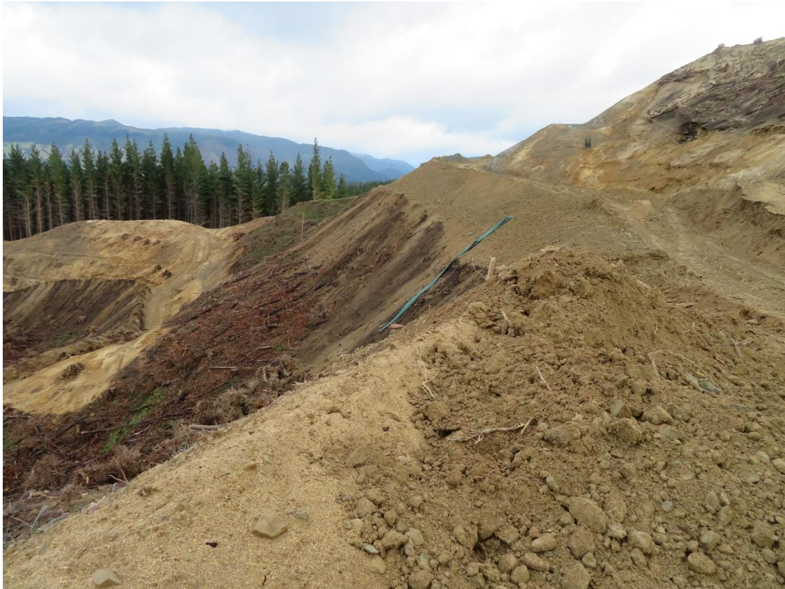
Photo 1: Pilot track to Landings 42 and 44.
