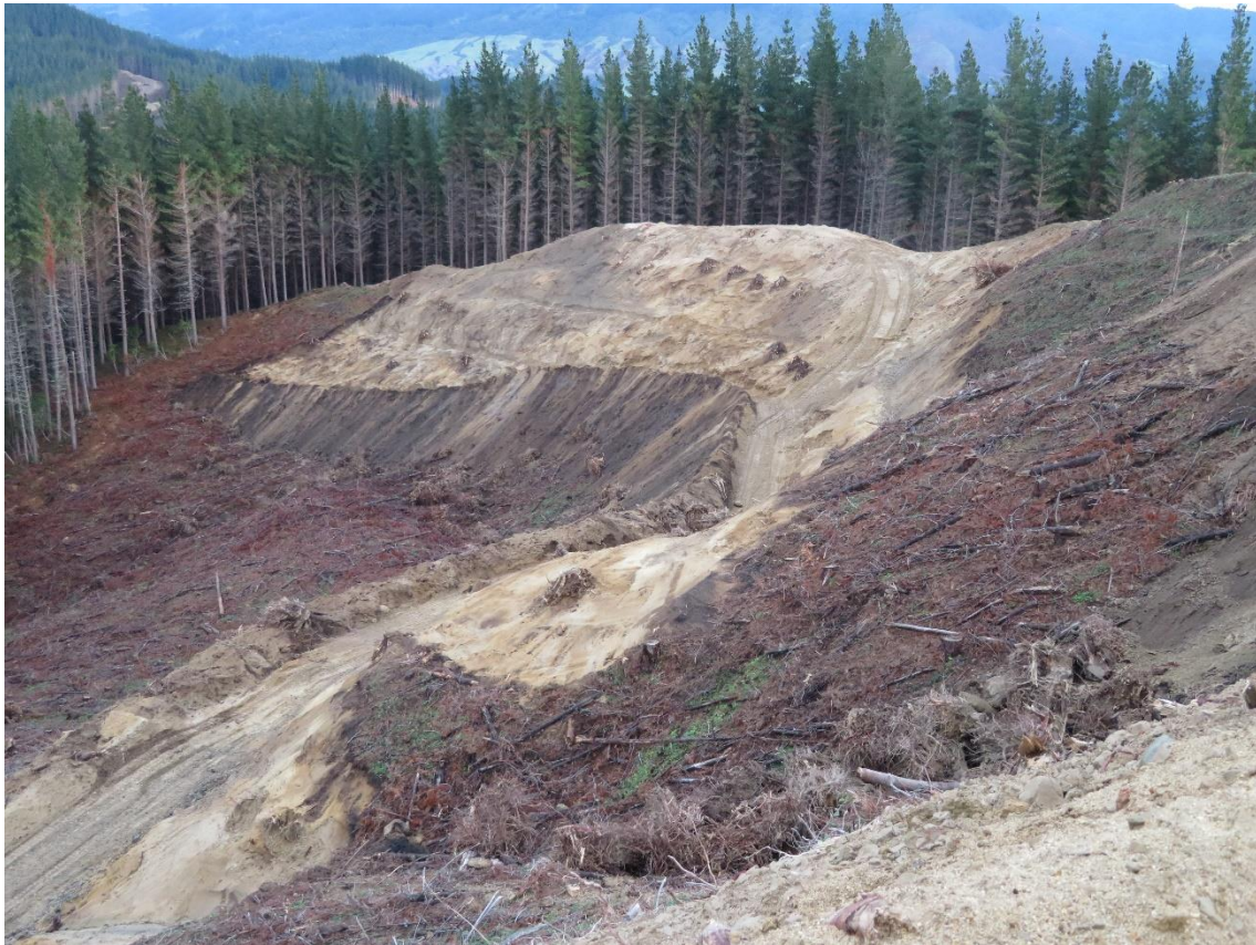
Photo 2: Topsoil stripped off soon to be constructed Landing 44.
