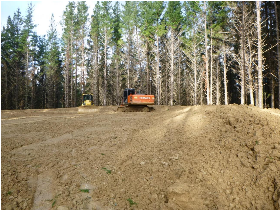
Photo 6: Tahurua Earthmovers enlarging Pad 16 at the end of Dixon Road.
