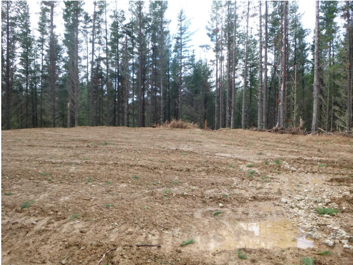
Photo 7: Pad 15 at the end of McIntosh Road - enlarged by Tahurua Earthmovers.
