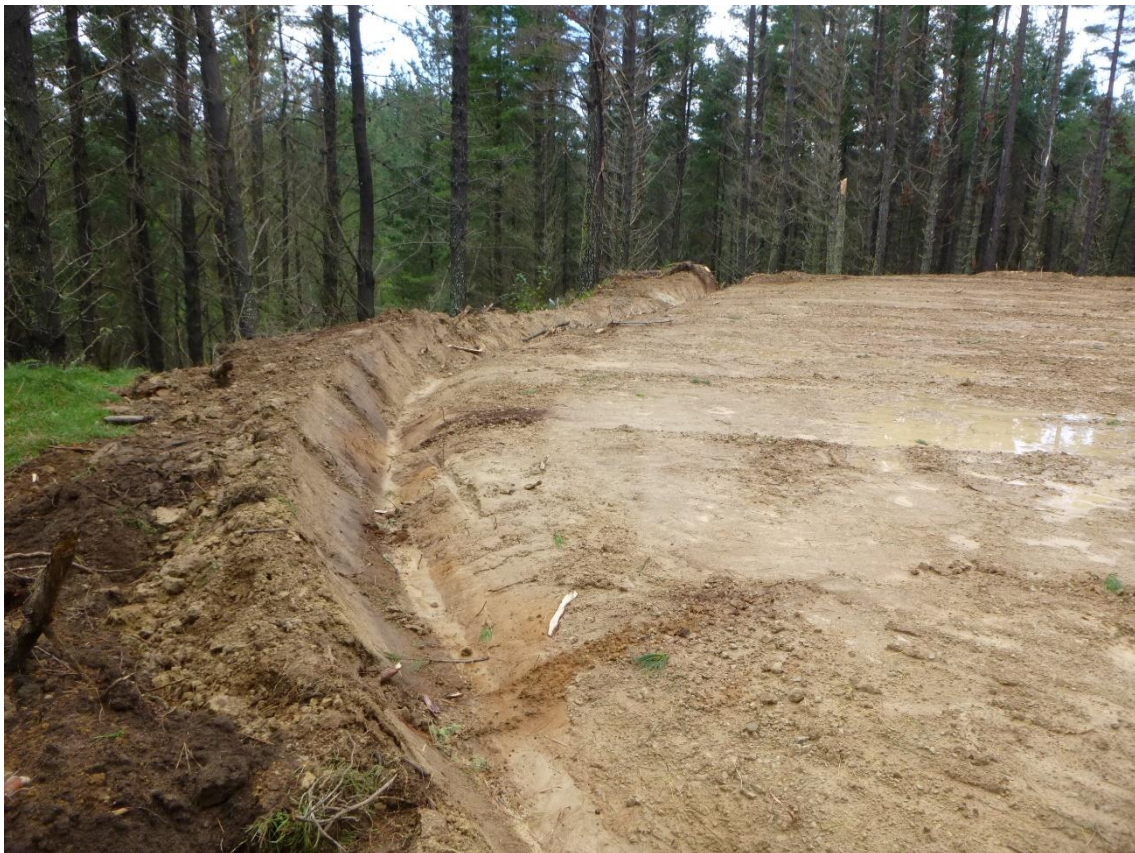
Photo 8: Pad 15 at the end of McIntosh Road - enlarged by Tahurua Earthmovers.
