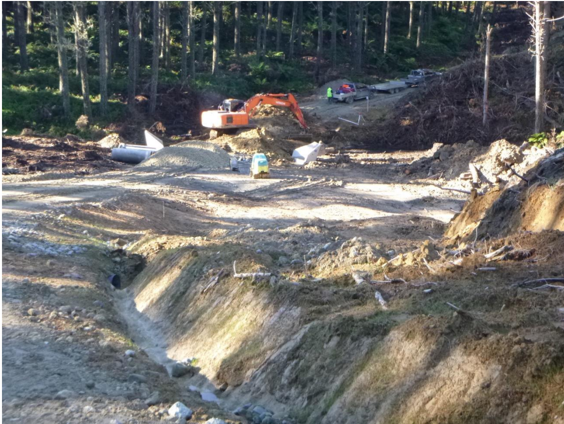
Photo 3: Tahurua Earthmovers installing crossing 5 on Rolfe Road.
