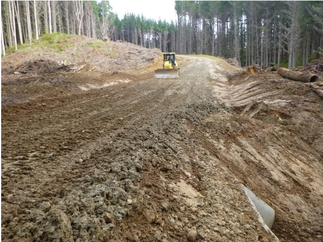
Photo 5: Tahurua Earthmovers forming Rolfe Road above crossing 5.
