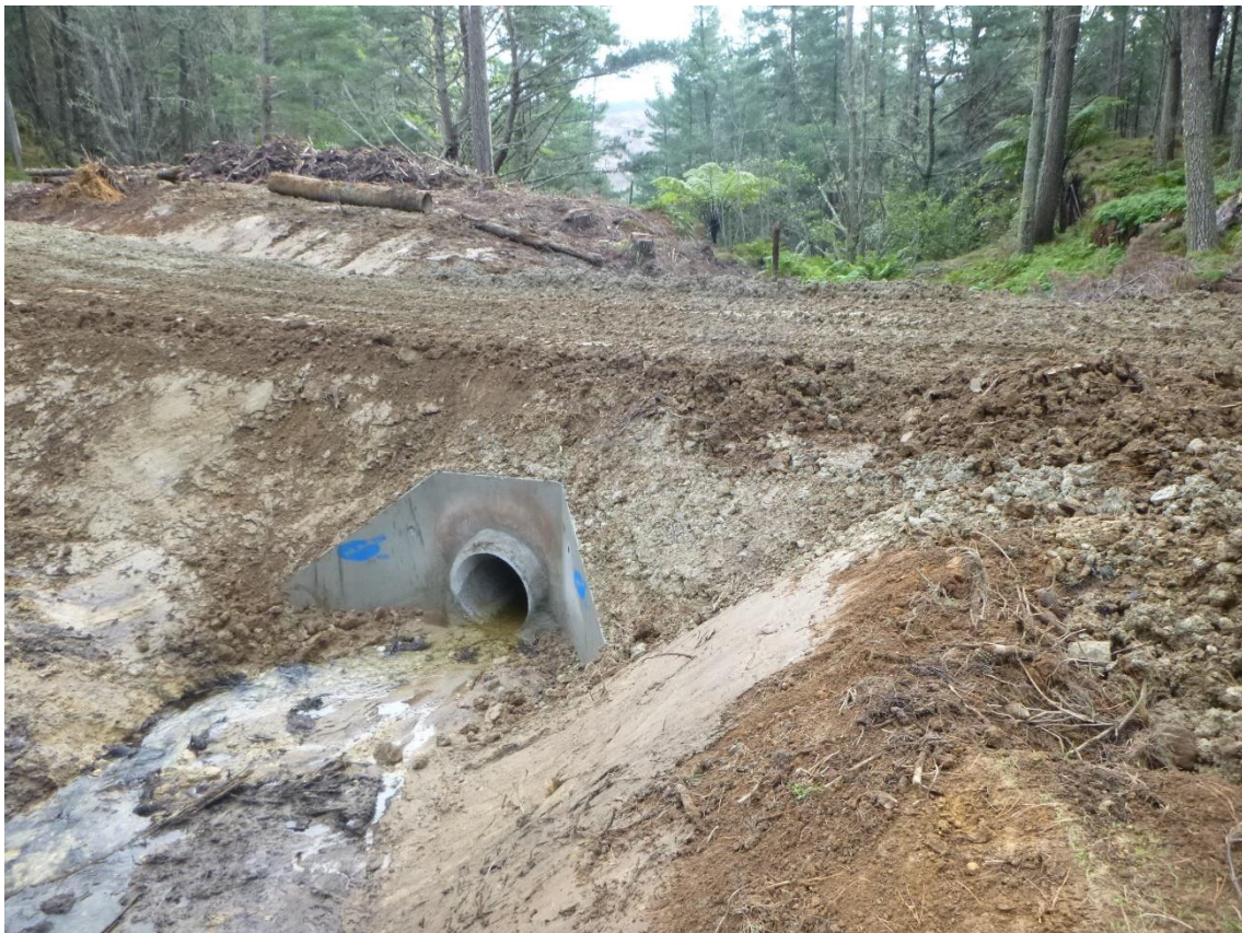
Photo 4: Crossing 5 installed by Tahurua Earthmovers on Rolfe Road.
