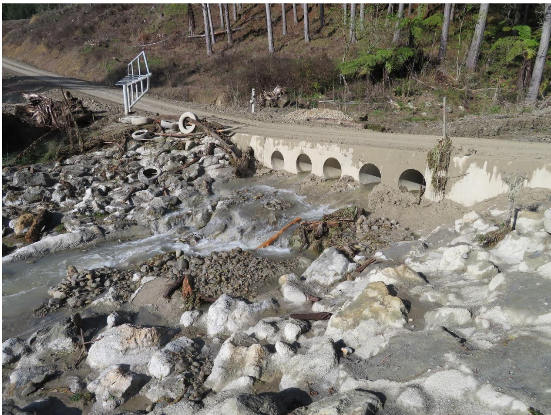
Photo 2: Battery concrete ford crossing Richmond Rd, access for all Ruakituri Forests.
