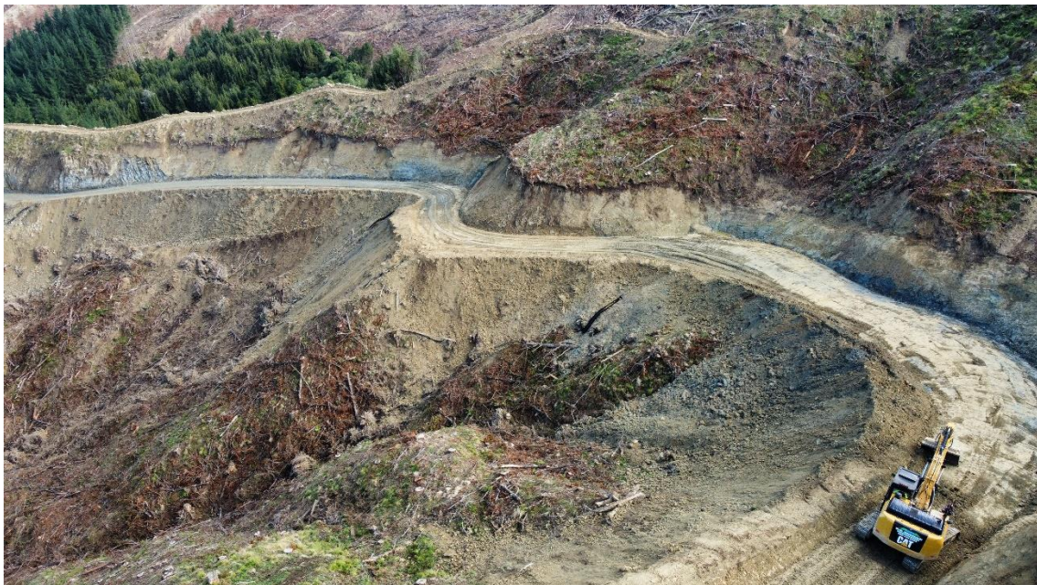
Photo 4: Excavator shaping Francis Road.
