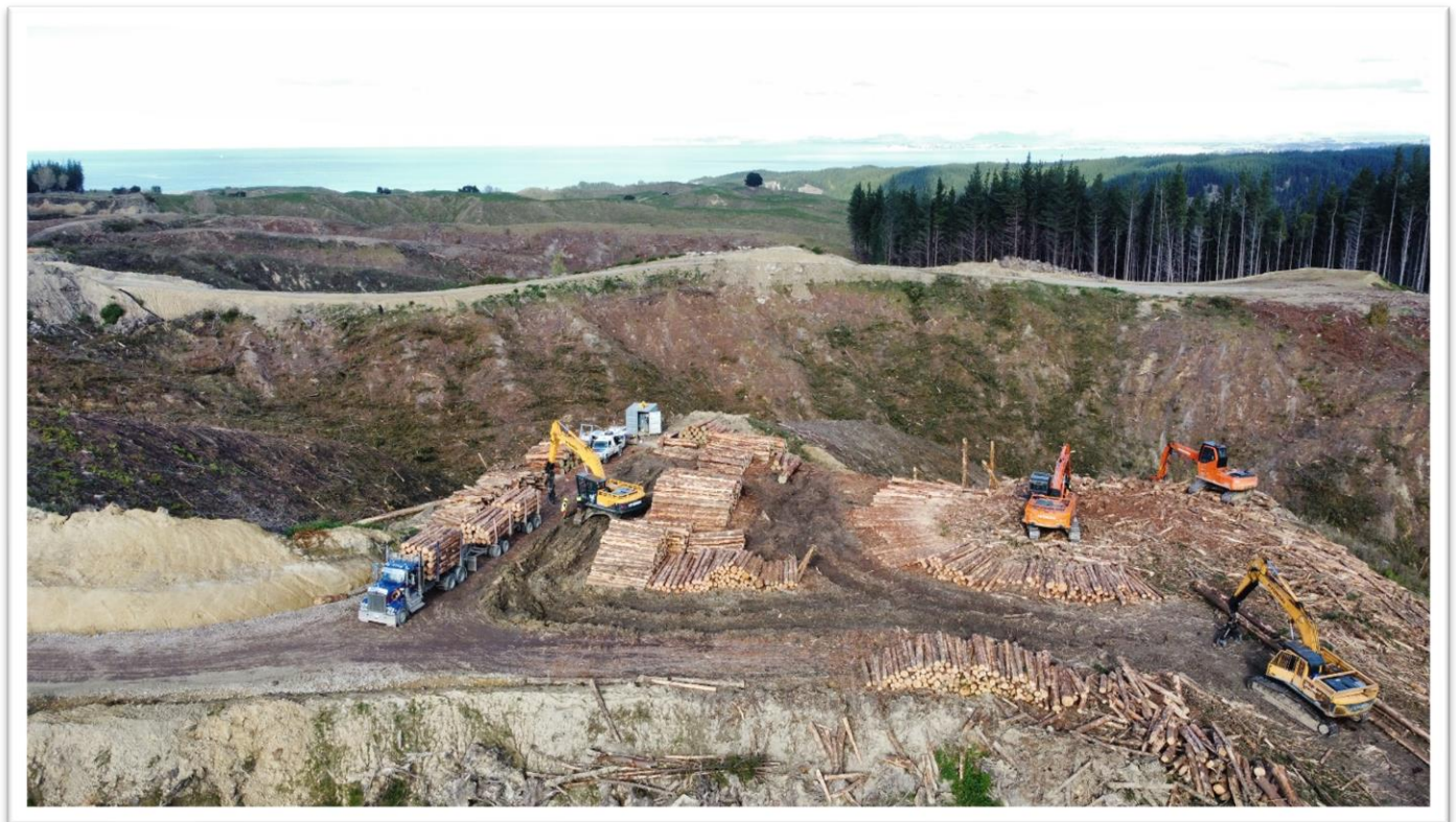
Log 12 operations in Setting 30, Napier in the background.
