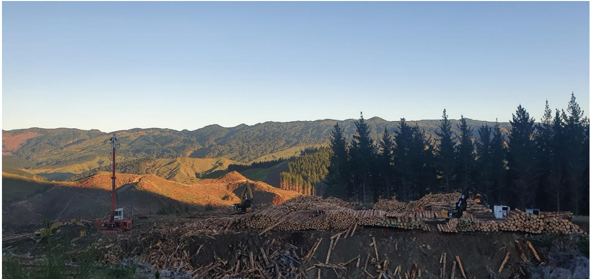
Photo 1: Clearfell crew working on Landing 82.
