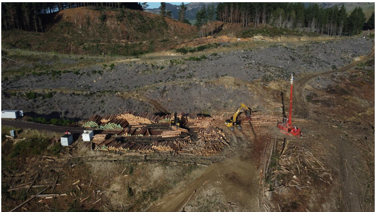
Photo 4: Clearfell crew working on landing 82.
