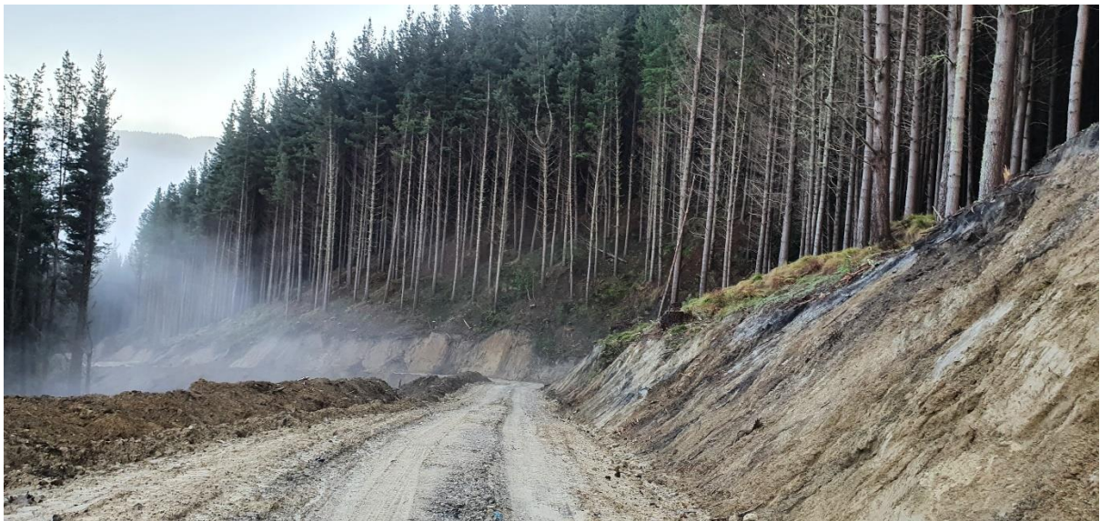
Photo 4: Aitken Road after roadline salvage.
