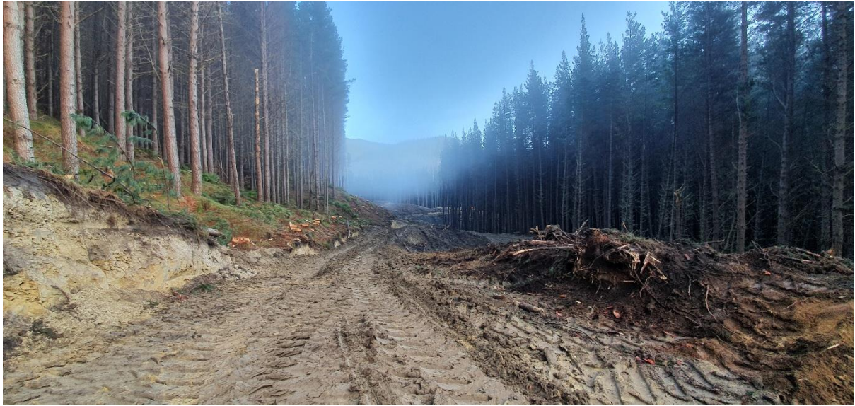
Photo 3: Roadline salvage of Aitken Road.
