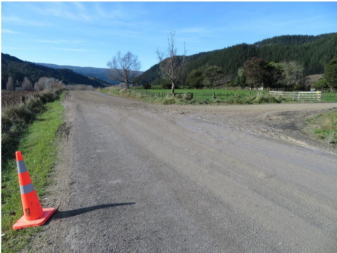
Photo 2: Entranceway onto public Ruakituri Road.
