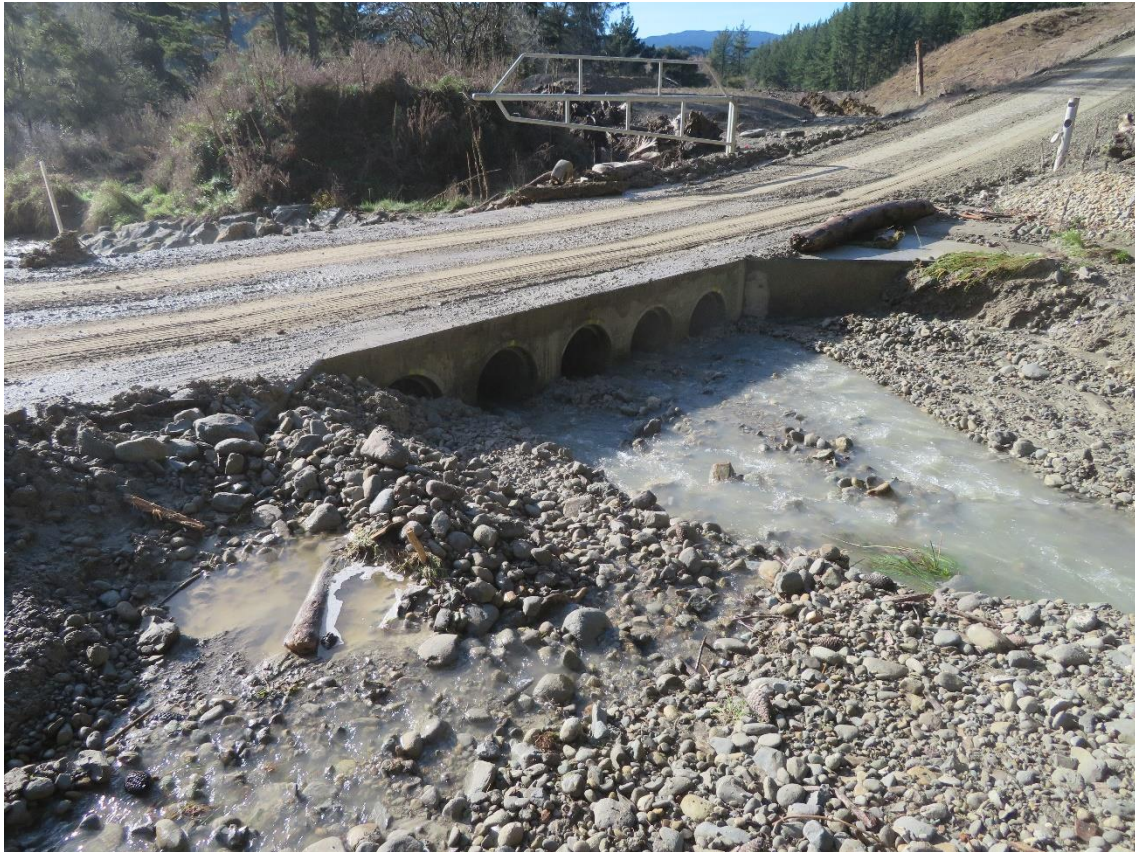
Photo 1: Battery concrete ford crossing on Richmond Road, access for all forests in the Ruakituri group.
