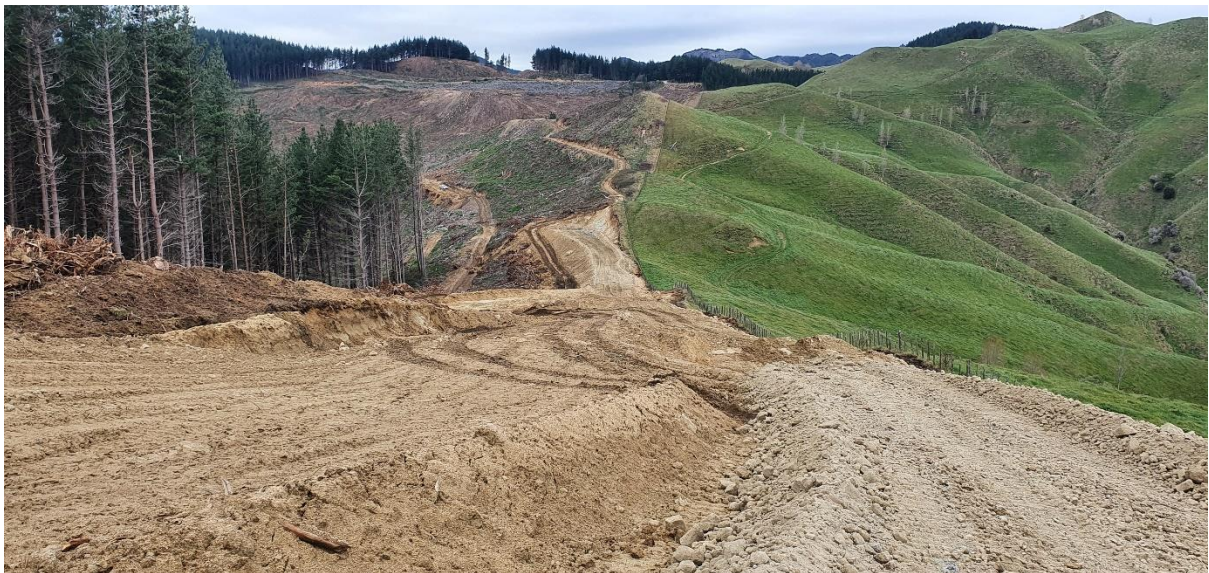
Photo 8: Adams Road under construction.
