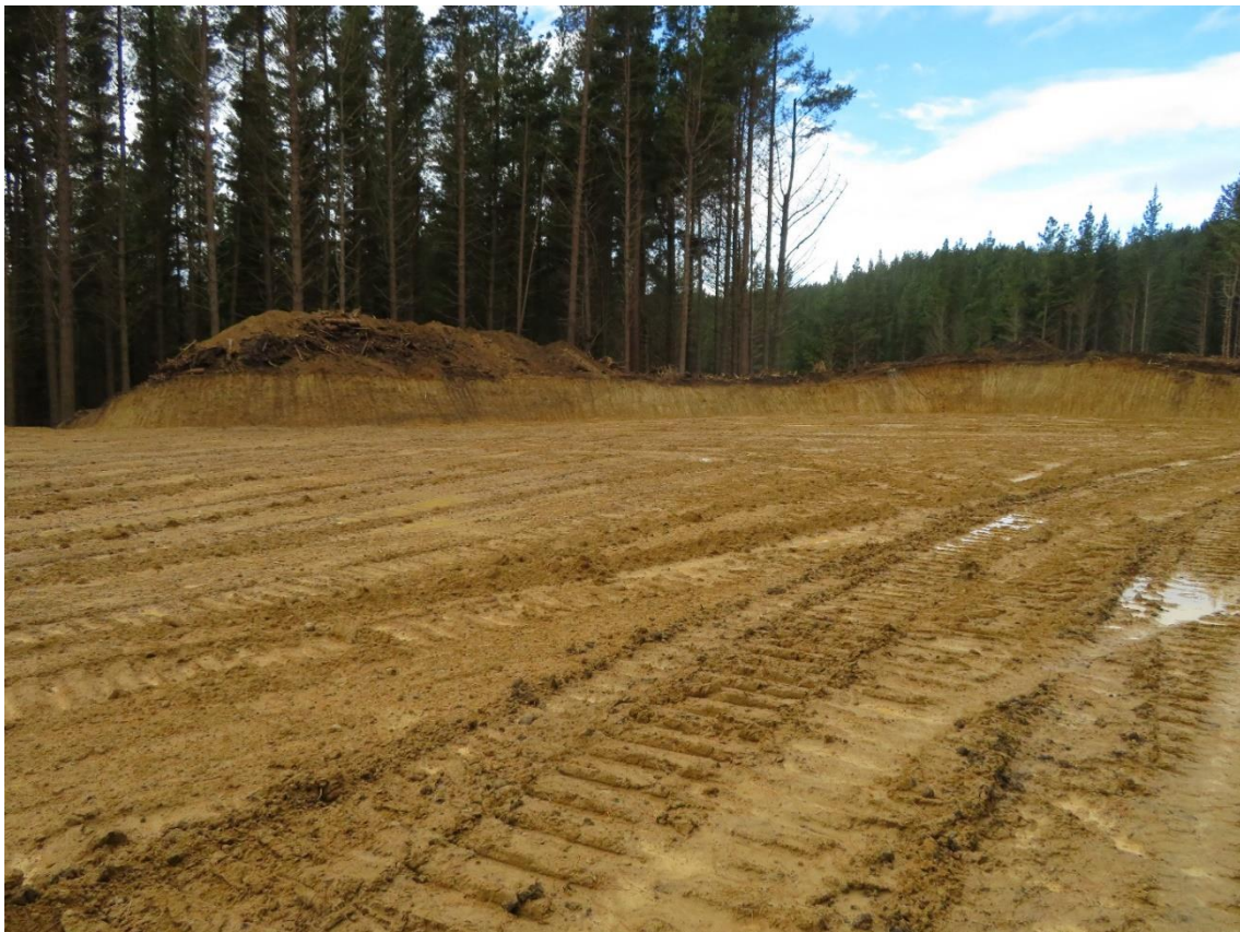
Photo 2: Recently constructed Landing 7.
