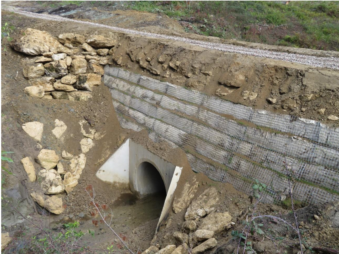
Photo 1: Griffiths Road permanent culvert crossing with Cirtex Duramesh to enable steeper fill face construction.
