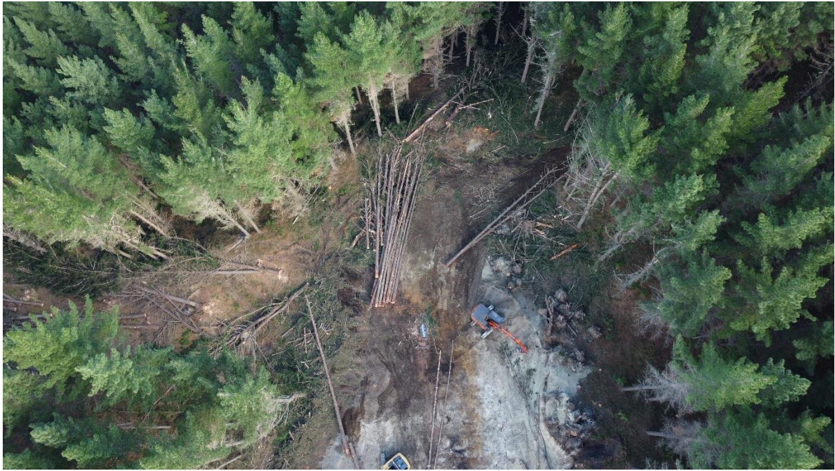
Photo 5: Siobhan Road roadline being felled and extracted.
