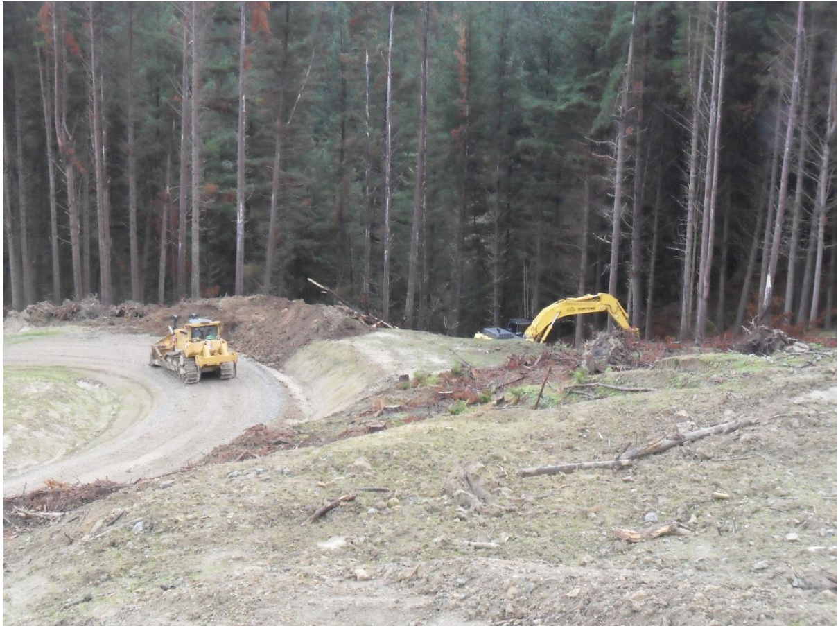
Photo 3: Pad being built to roadline Setting 508.
