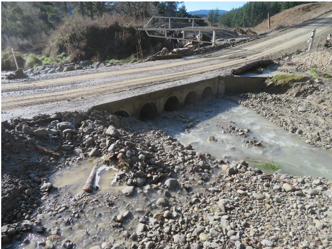
Photo 2: Battery concrete ford crossing on Richmond Road.
