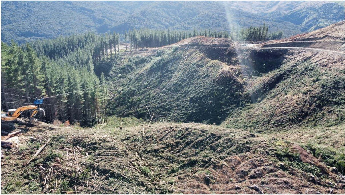
Photo 5: Hauler ropes across Setting 8.
