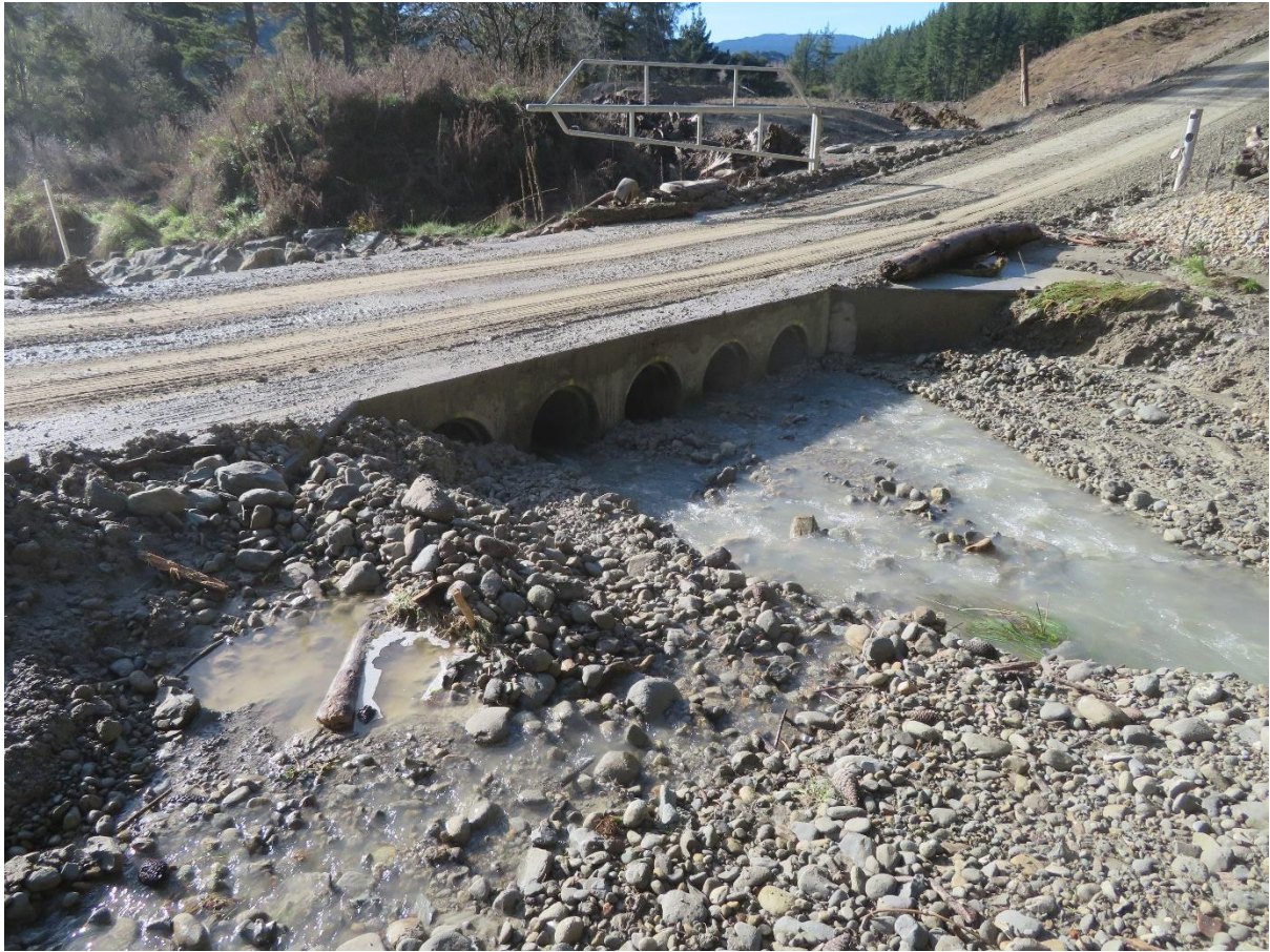
Photo 1: Battery concrete ford crossing Richmond Road, access for all forests in the Ruakituri Group.
