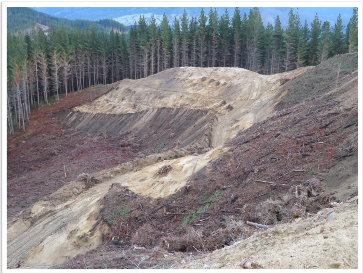
Landing 44 with topsoil stripped, ready for construction.
