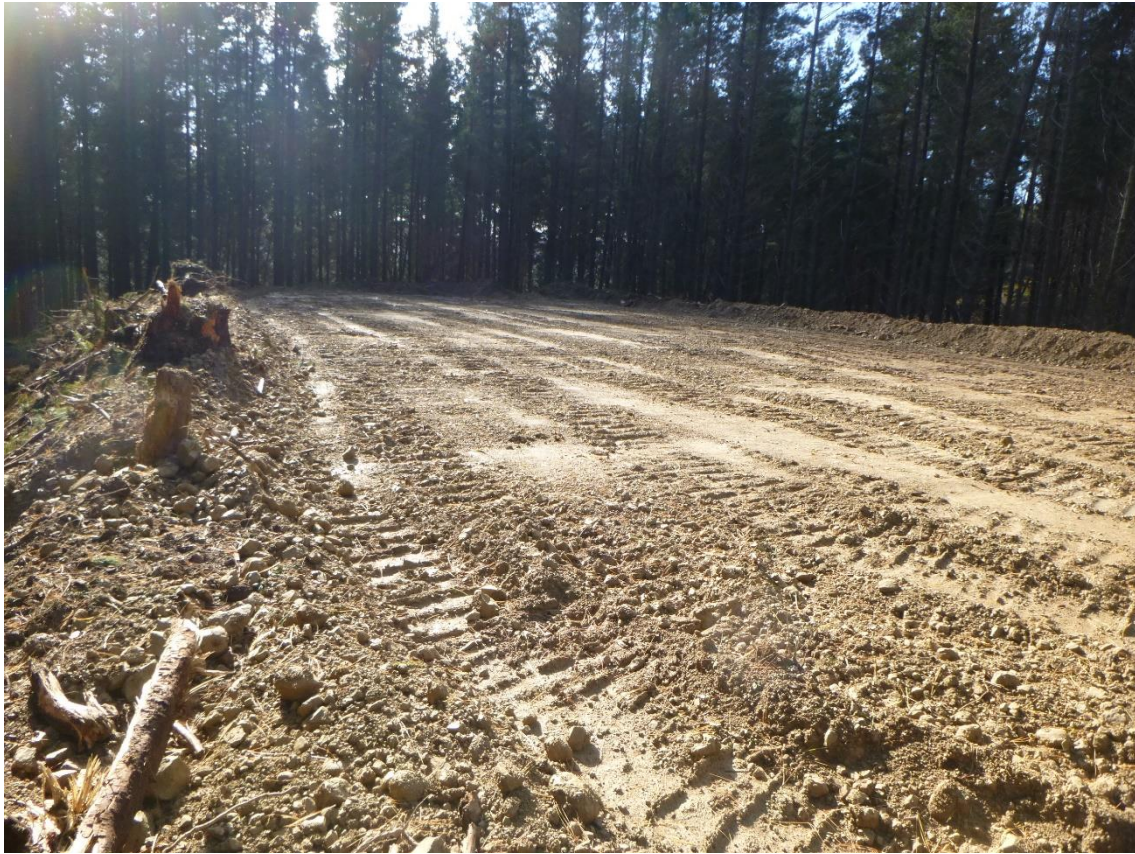
Photo 3: Tahurua Earthmovers partially constructed Pad 23 at the end of Rolfe Road.
