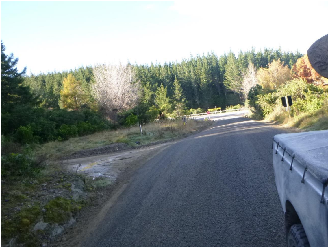
Photo 6: Recently chip sealed intersection between Tarewa Road and State Highway 2.
