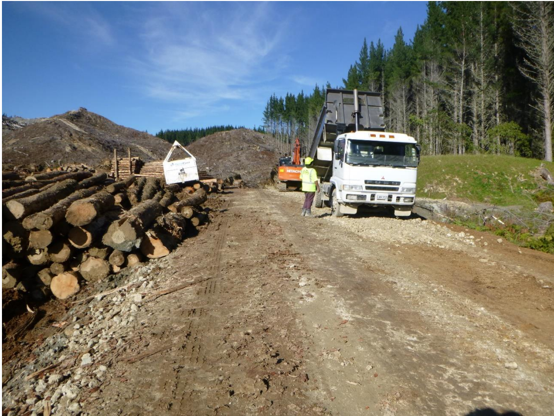
Photo 5: Tahurua Earthmovers metalling the loadout bay and turnaround for Ultimate Logging on Pad 5, Rolfe Road.
