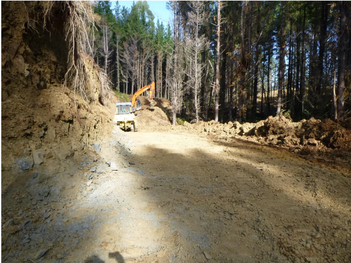
Photo 1: Tahurua Earthmovers constructing Rolfe Road between Pads T3 and 23.
