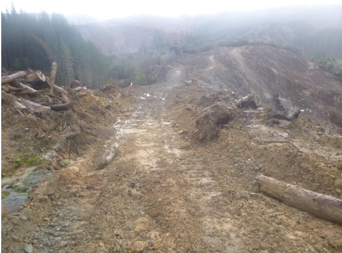
Photo 4: Tahurua Earthmovers - rehabilitation of quad track through Setting 8, opening access for the replanting crews.
