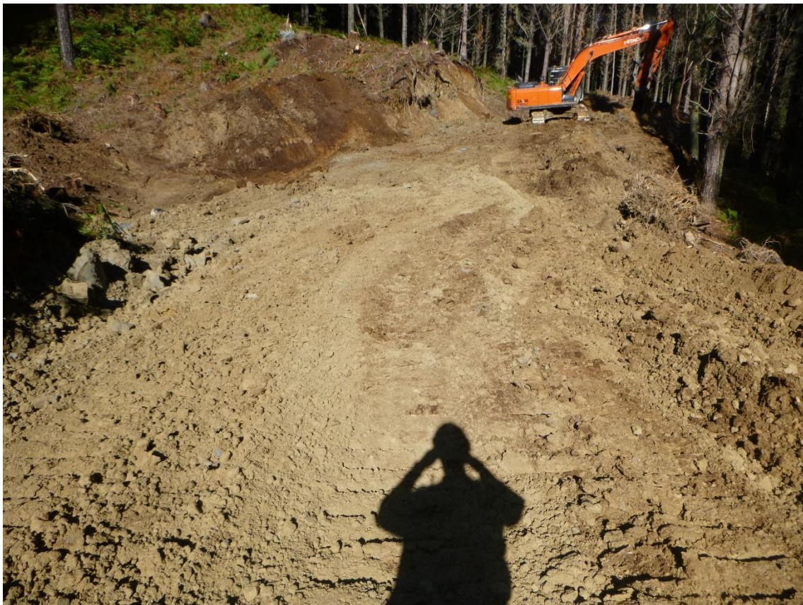
Photo 2: Tahurua Earthmovers constructing Rolfe Road between Pads T3 and 23, installing culverts.
