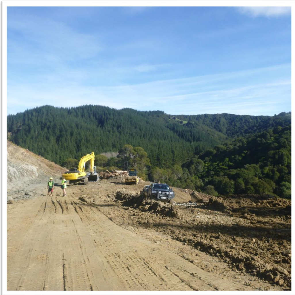
Maloy Road construction on the lower section of the road towards the crossing.
