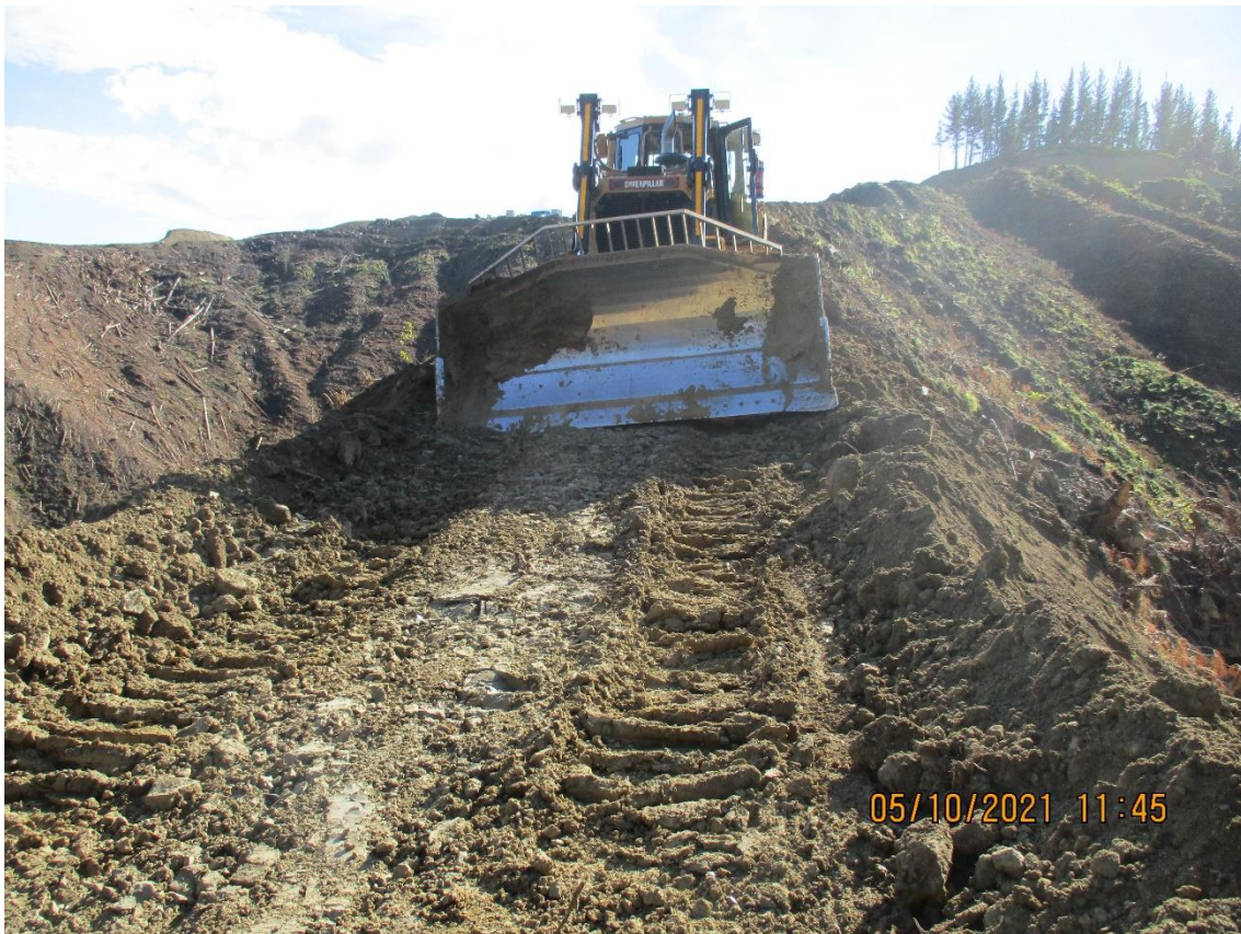
Photo 2: Bulldozer coming down a pilot track.
