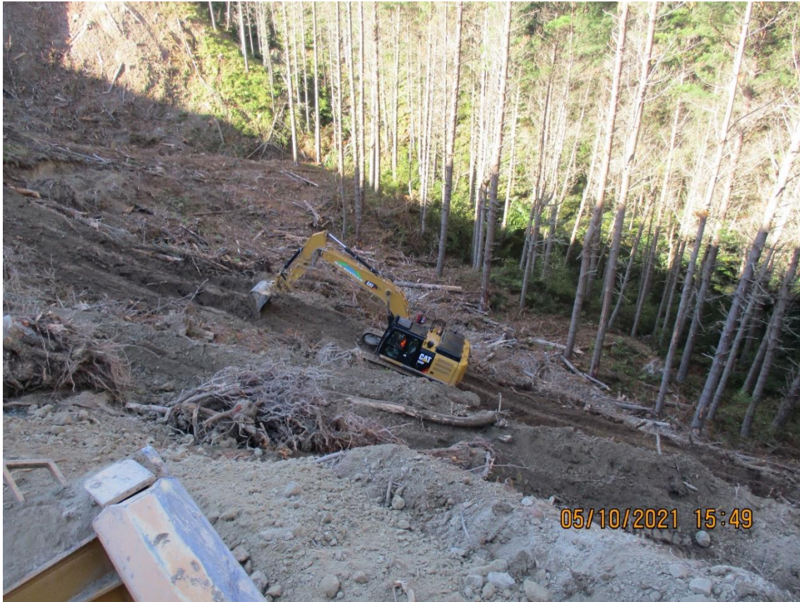
Photo 3: Excavator benching Landing 605 for fill.
