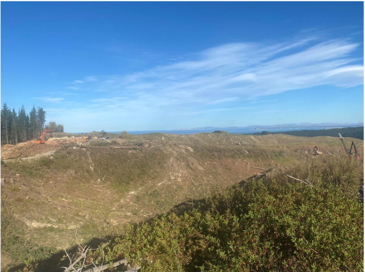
Setting 49 viewed from T9, the swing yarder operating from a two-stage pad and processing on 49.
