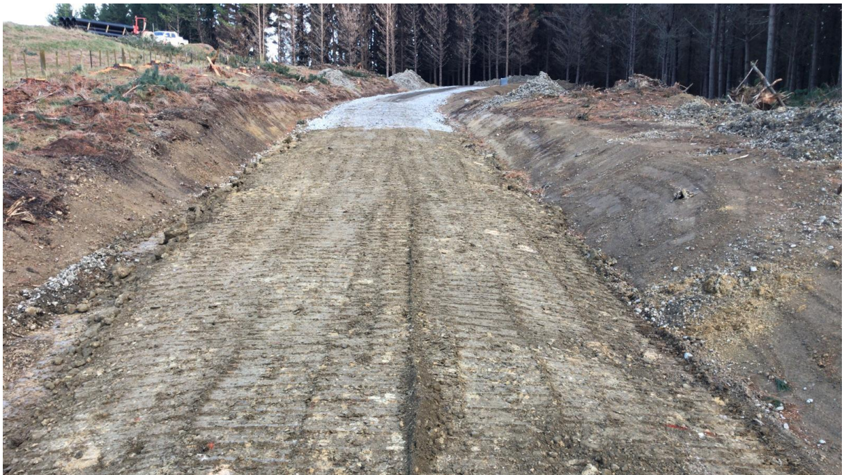
Photo 4: Red metal on the road to the airstrip.
