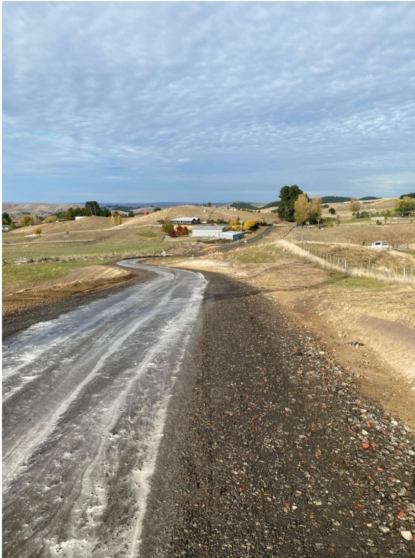
Photo 1: Dust suppressant applied at the entrance of Kiwiroa Road.
