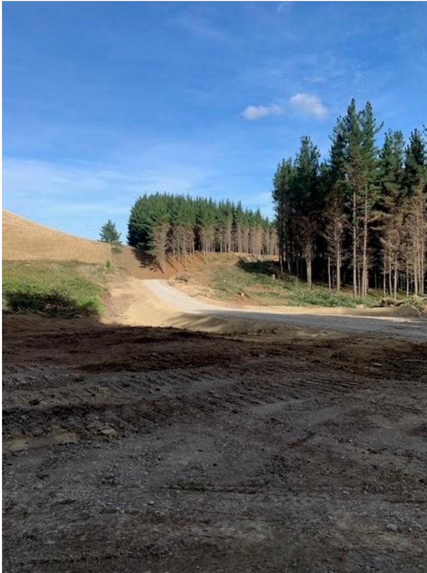
Photo 5: Newly formed section of Tutaekuri Road.
