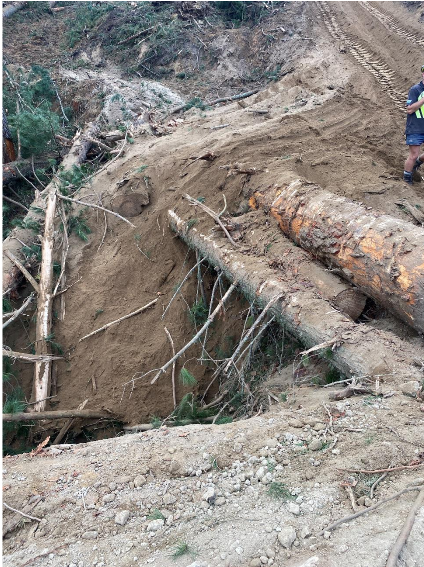
Photo 6: Logs used to support a temporary stream crossing between Landings 24 and 25.
