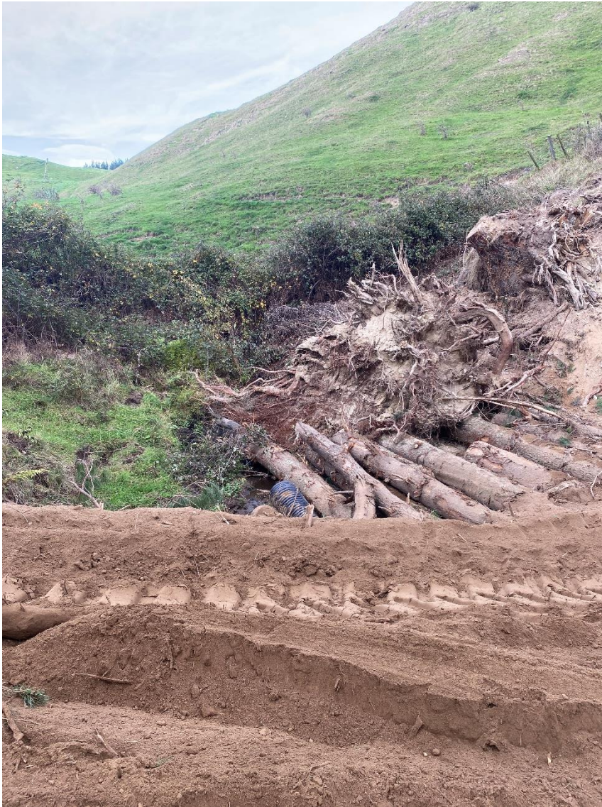
Photo 5: Temporary stream crossing in place for machinery to cross between Landings 24 and 25.
