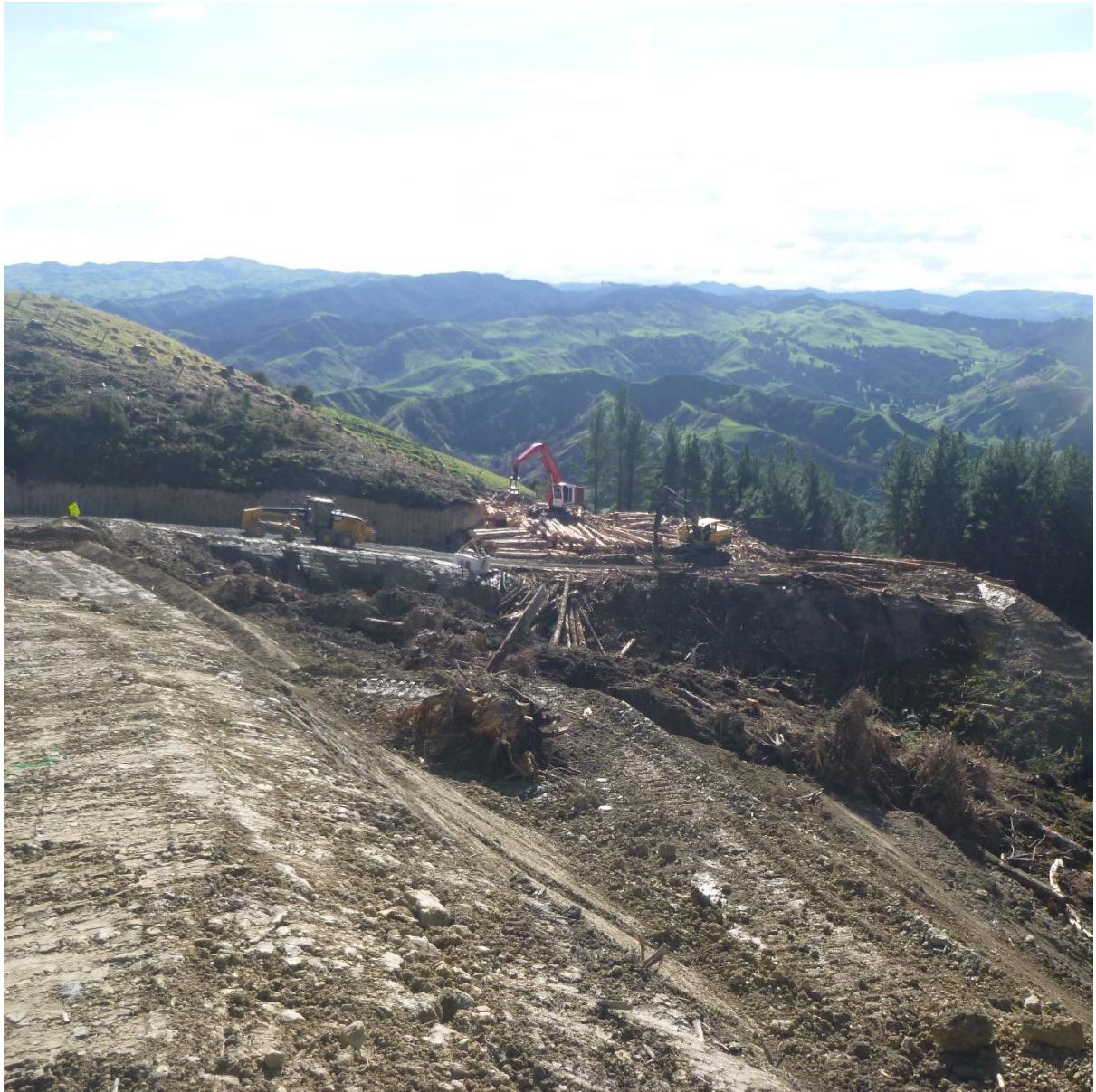
Photo 3: Overlooking operations on Pad 13.
