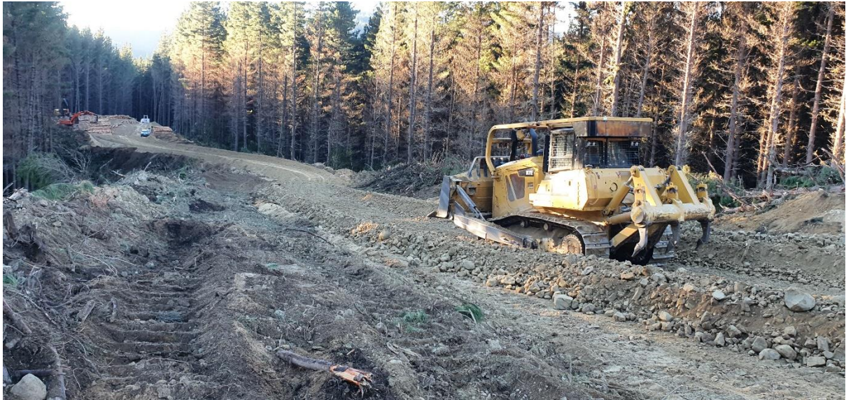
Photo 1: Bulldozer forming the road to Landing 104.
