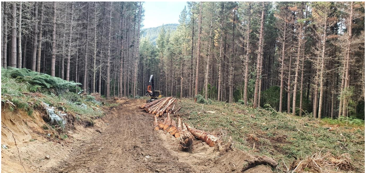
Photo 6: Falling machine falling and shovelling stems on roadline from Landing 104 to 105.
