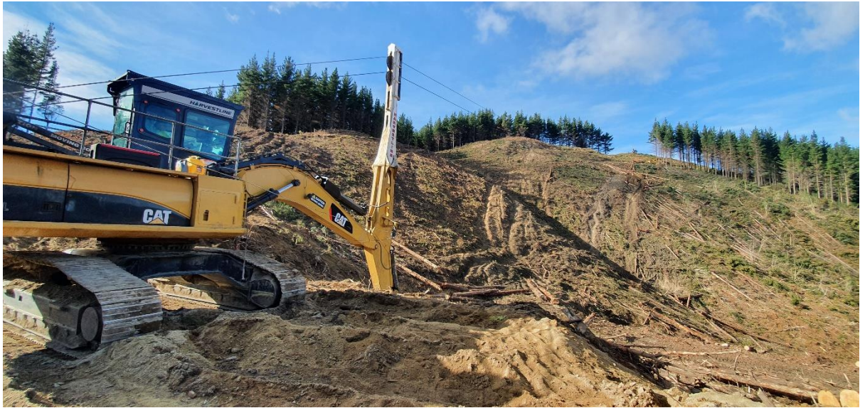
Photo 3: Log 7 harvestline extracting stems to Landing 145.
