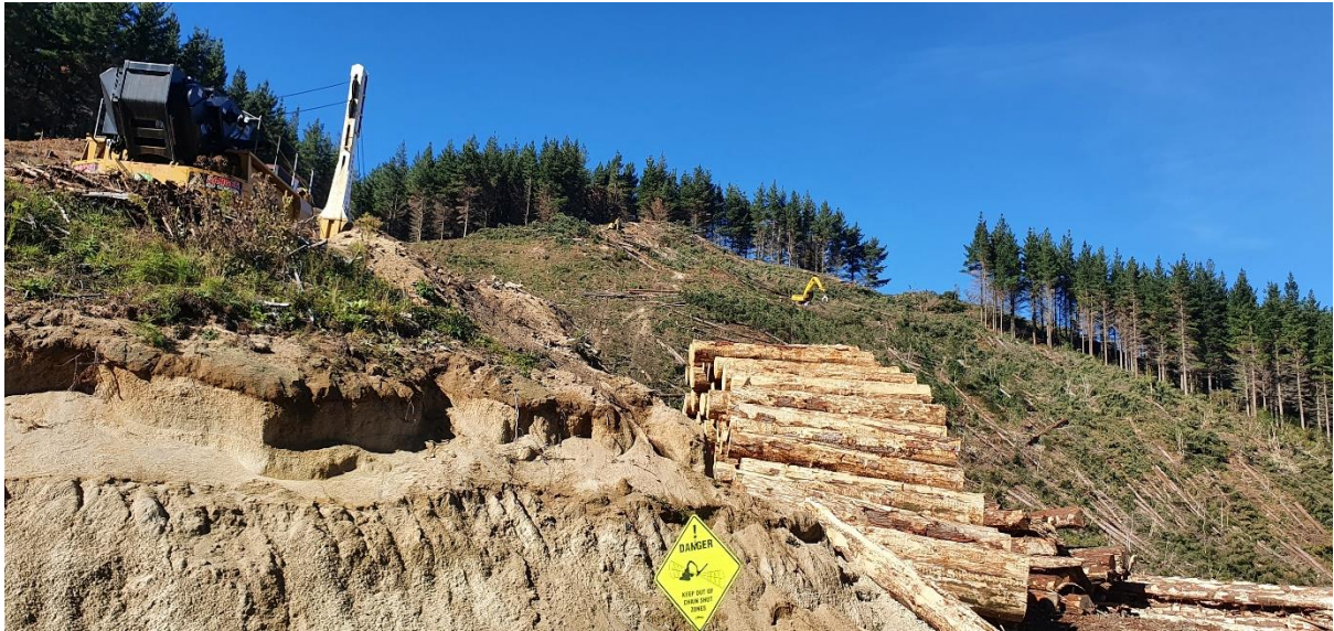
Photo 1: Log 7 harvestline extracting stems to Landing 145 with machine up the hill shovelling stems.
