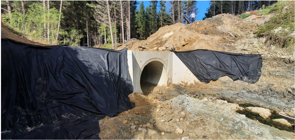
Photo 3: Geo cloth behind lime rock wingwall.
