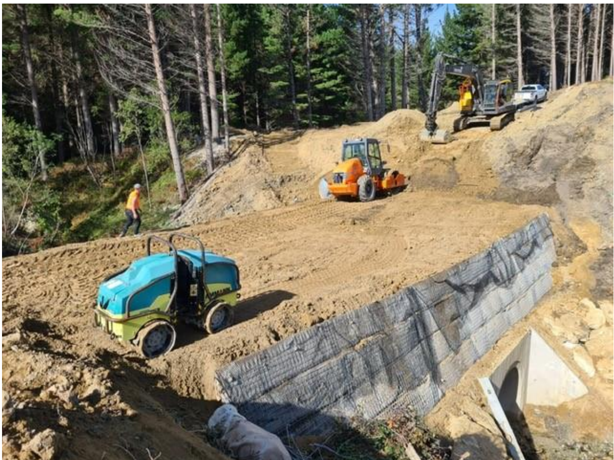
Photo 2: 2m crossing bank stabilisation.
