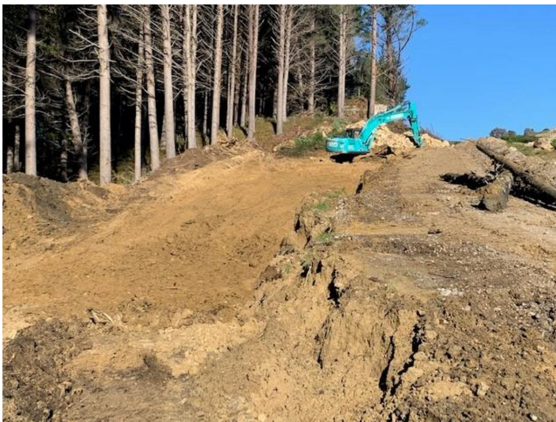
Photo 6: Constructing the road to the crossing.
