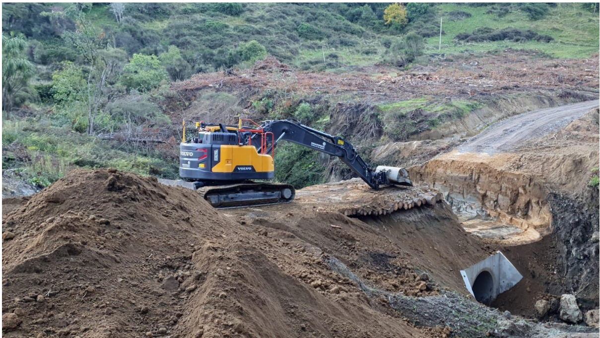
Photo 4: Installation of crossing.
