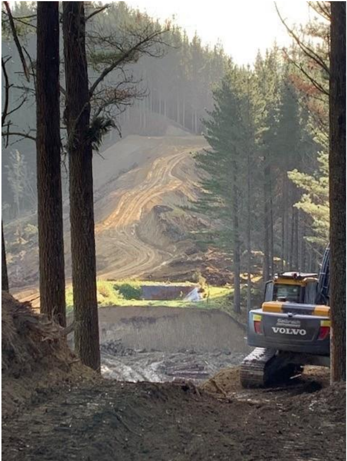
Photo 2: Newly formed road from Landing 29 to 30.
