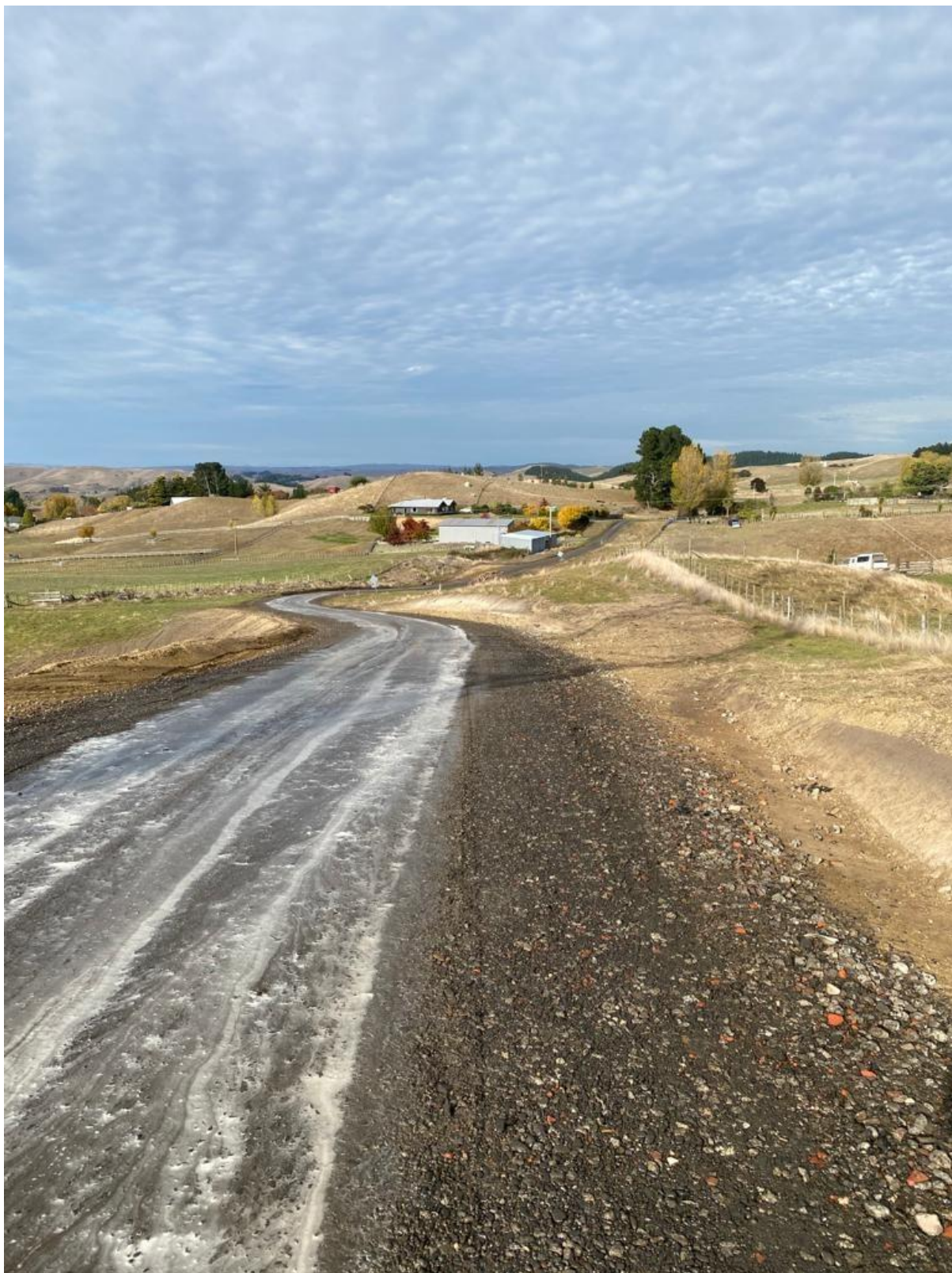
Photo 2: Dust suppressant applied at the entrance of Kiwiroa Road.
