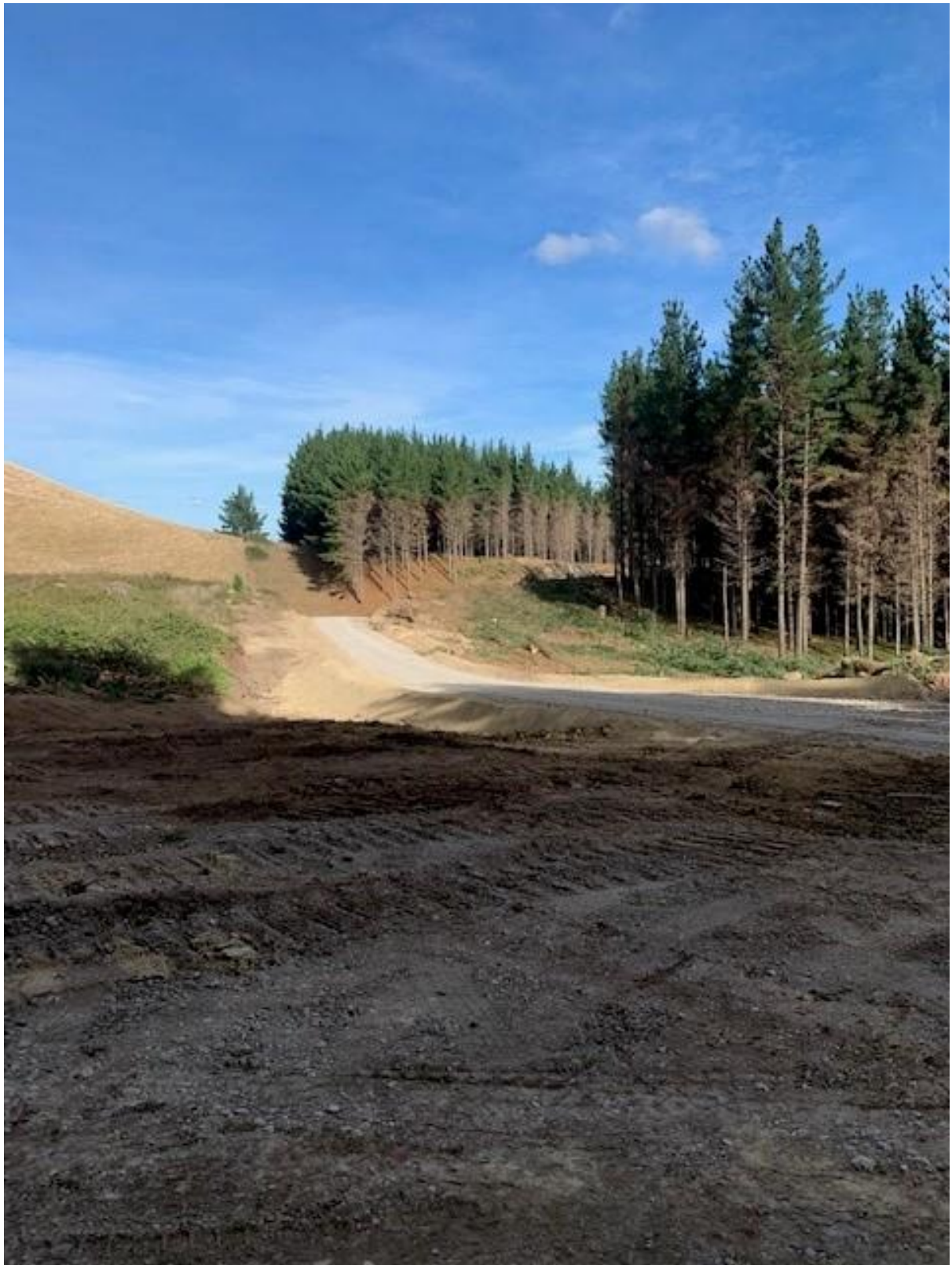
Photo 5: Newly formed section of Tutaekuri Road.
