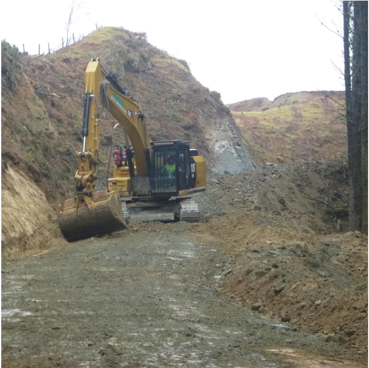
Photo 2: Setting up water bars for rain event coming in on Wairoa River Road.
