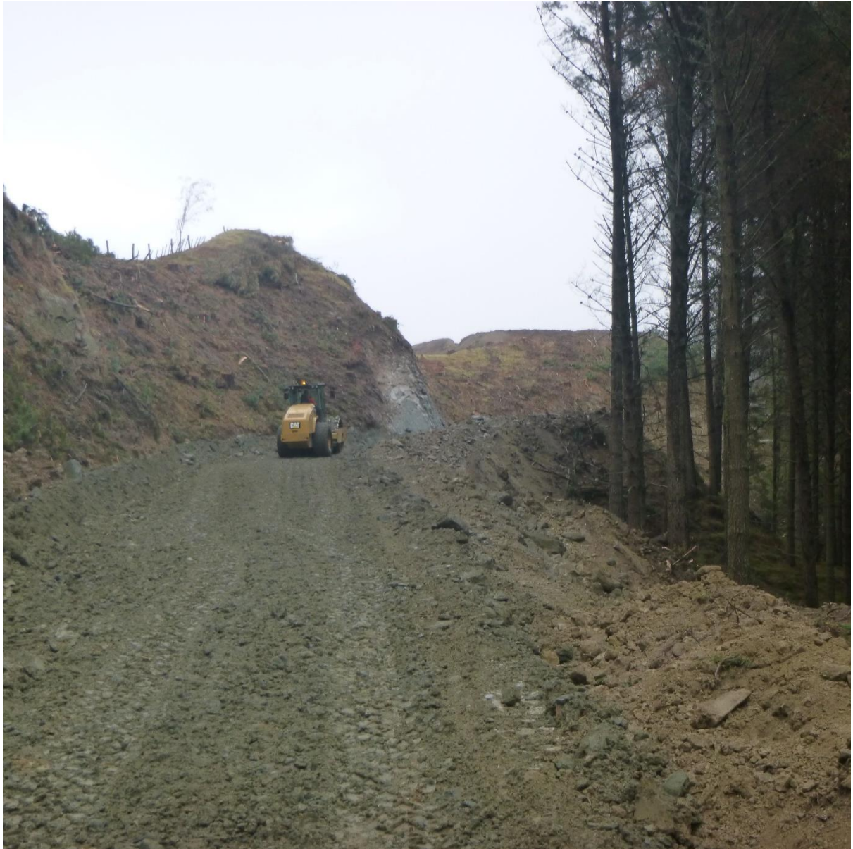
Photo 1: Compacting fill on Wairoa River Road.
